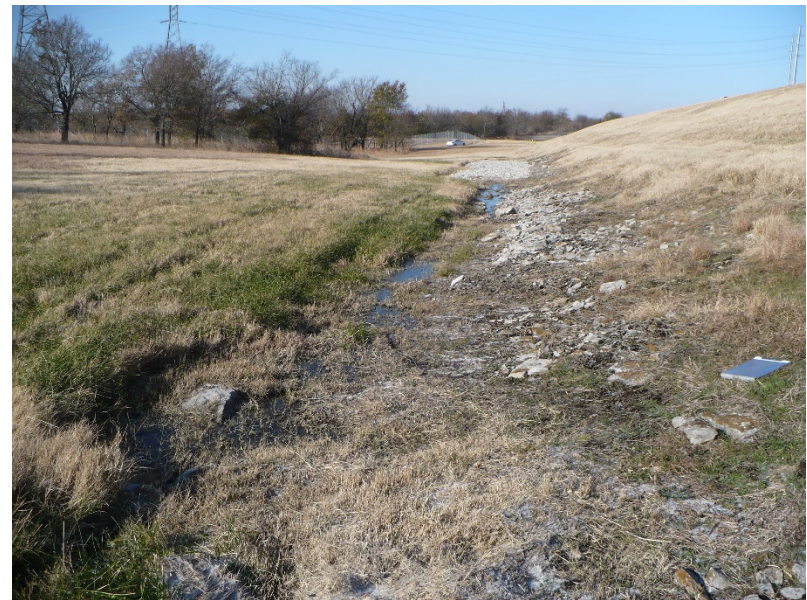
Photo #8 – toe of south dike-some ponded water in ditch
