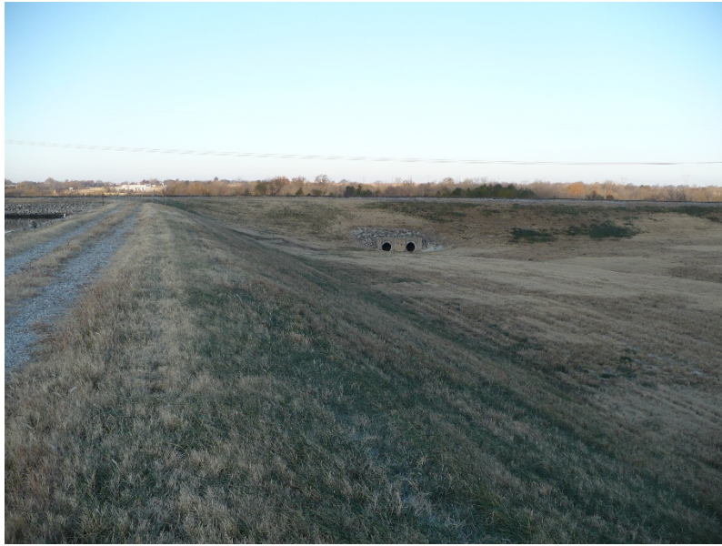
Photo #1 – exterior slope north dike– looking west
