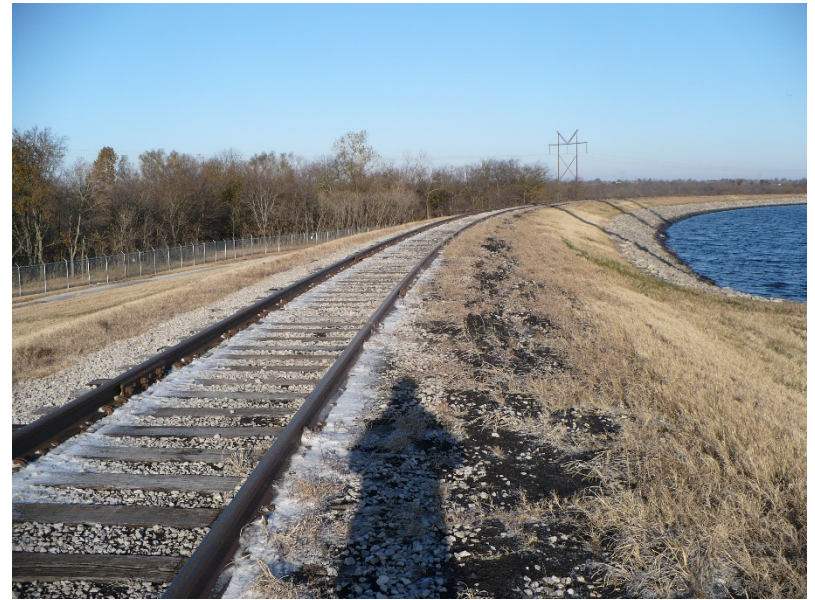
Photo #6 – crest of west dike
