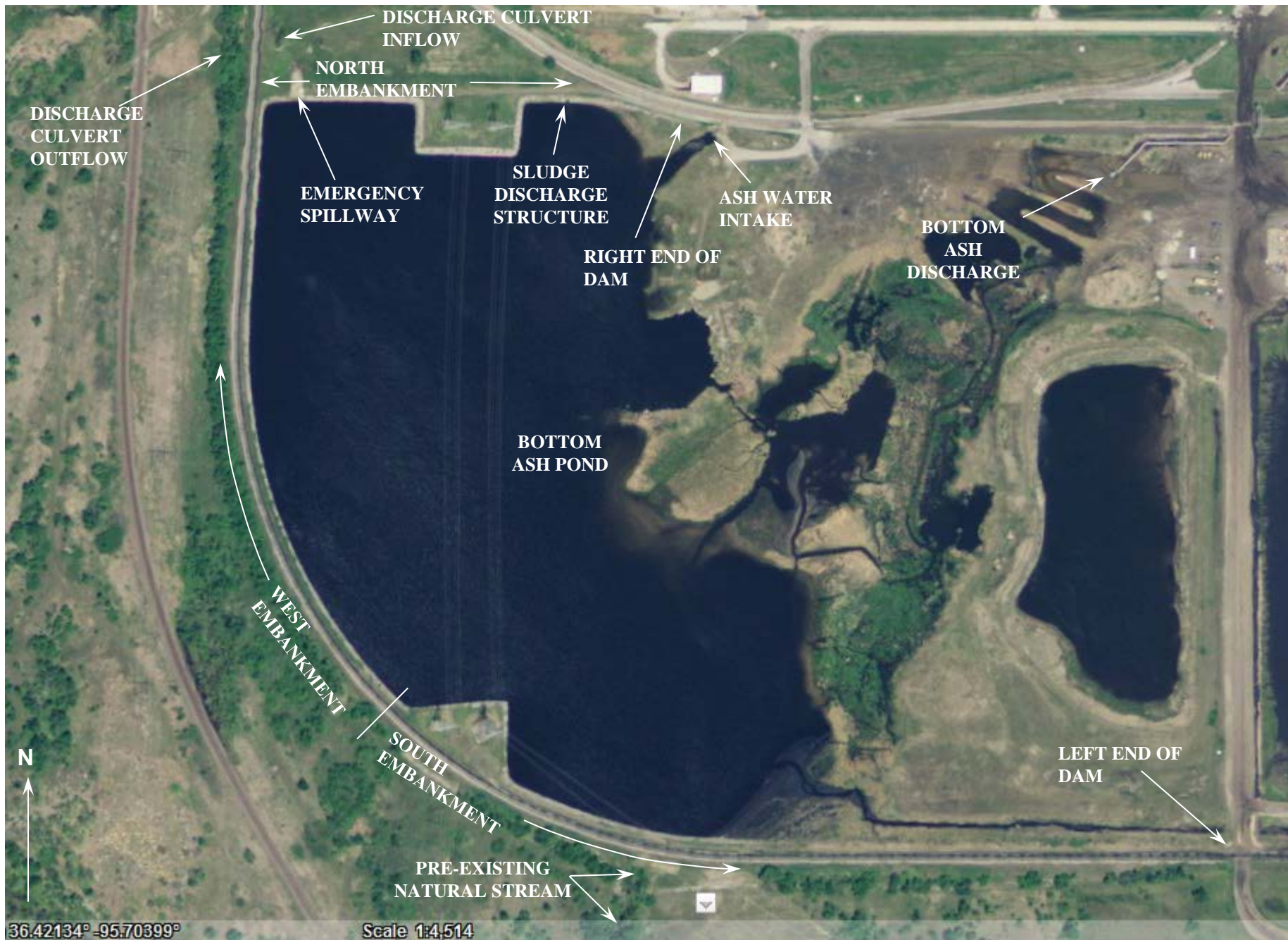
Figure 1. Satellite Image Of Bottom Ash Pond Dam, Features, And Appurtenances At Northeastern 3&4 Power Station.
