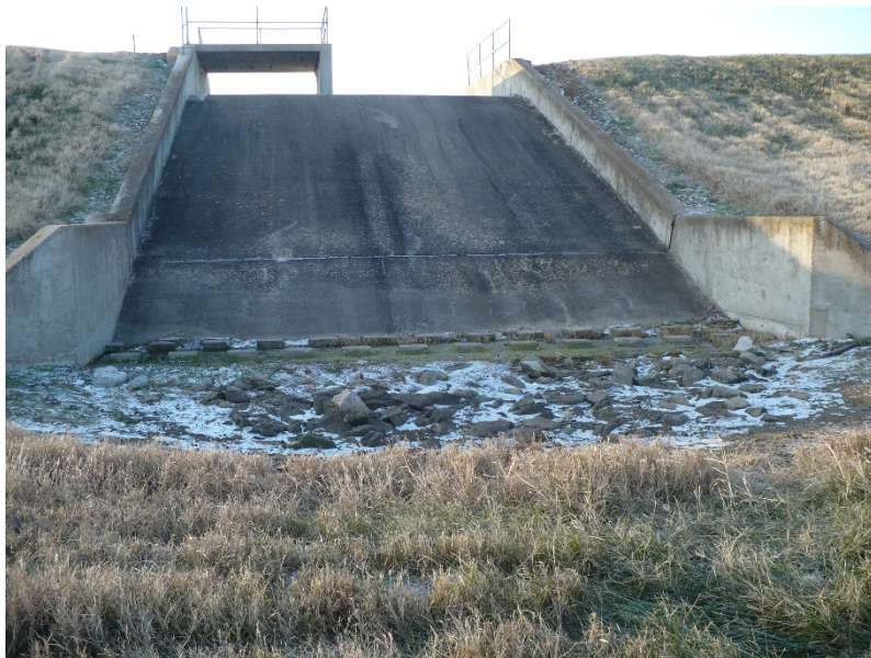
Photo #3 –spillway chute
