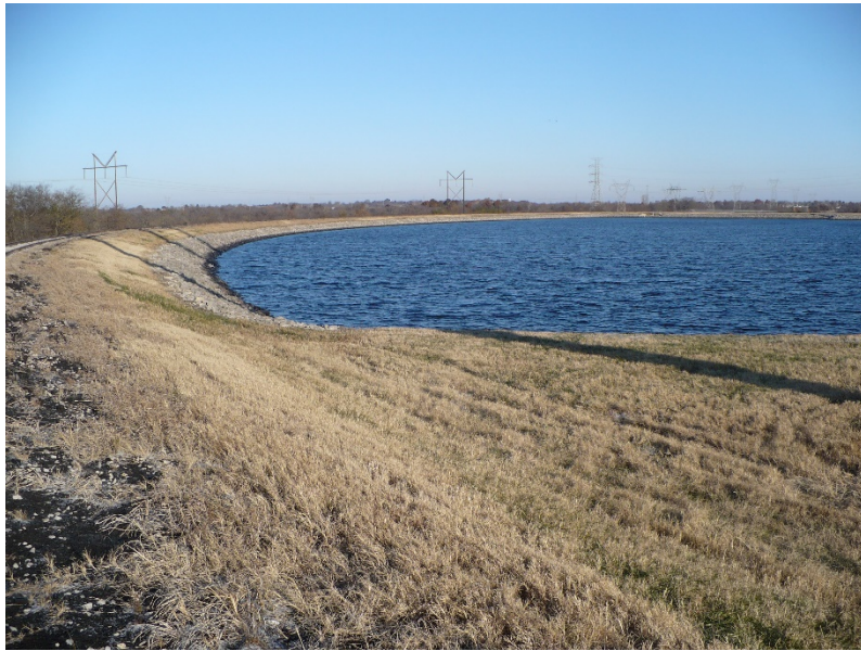
Photo #5 – interior slope of west dike
