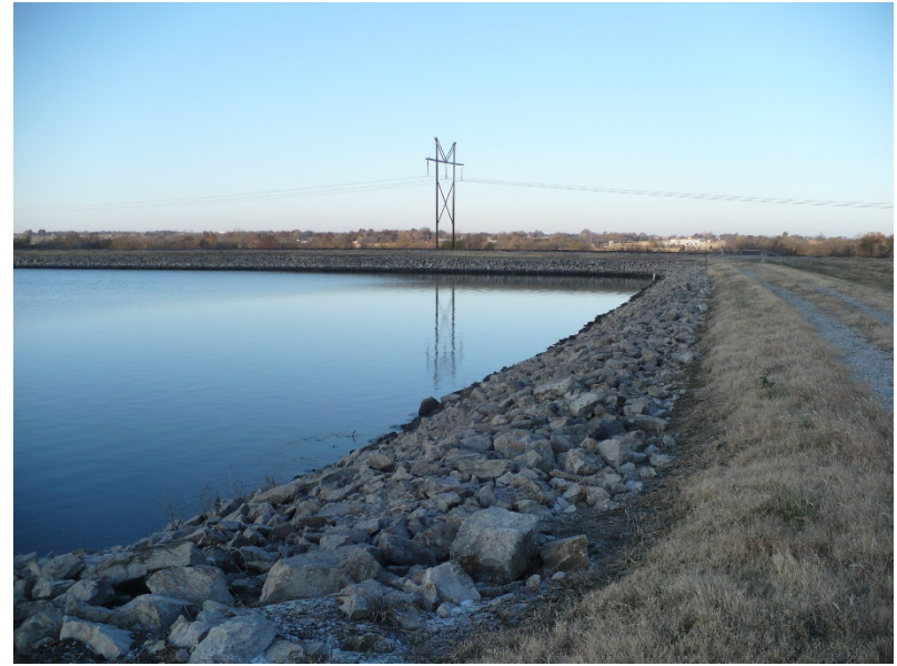
Photo #2 – interior slope of north dike-looking west
