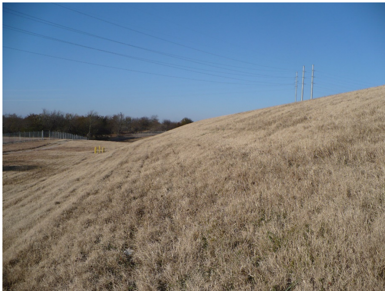
Photo #7 – exterior slope of south dike-looking west
