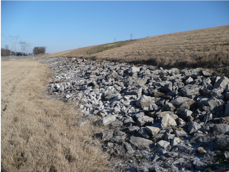
Photo #9 – exterior slope of west dike-looking north
