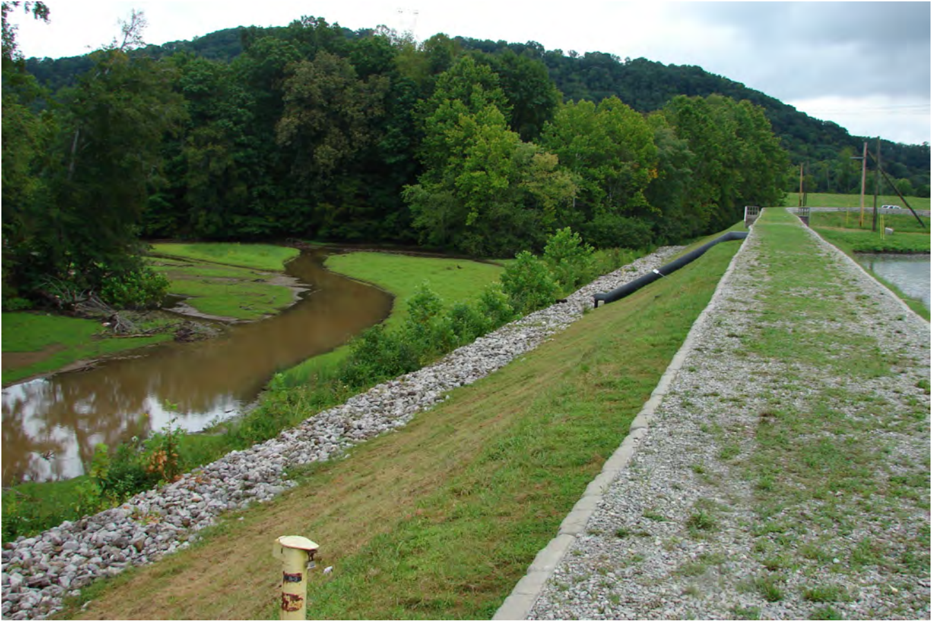
Photograph 3. Downstream Slope and Bills Creek.
