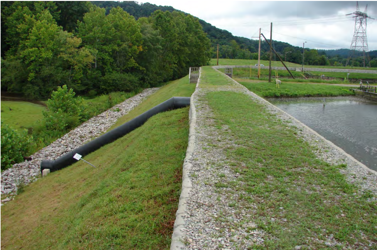
Photograph 2. Reclaim Pond Spillway Pipe and Downstream Slope.
