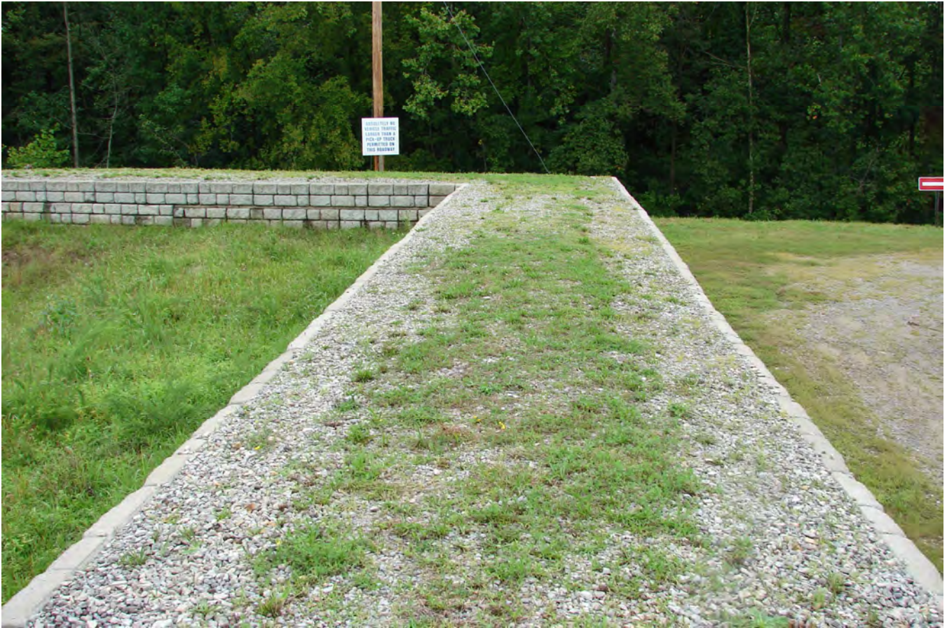
Photograph 4. Redi-rock Soil Reinforcement.
