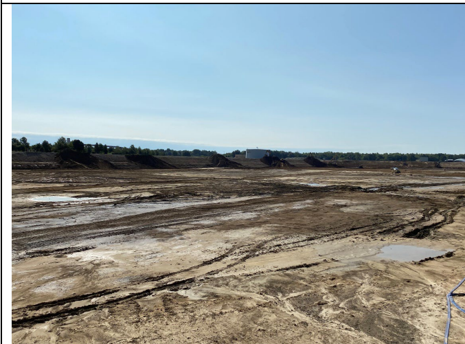
Photograph 9: #E View of the pond bottom of the East Bottom Ash Pond.
