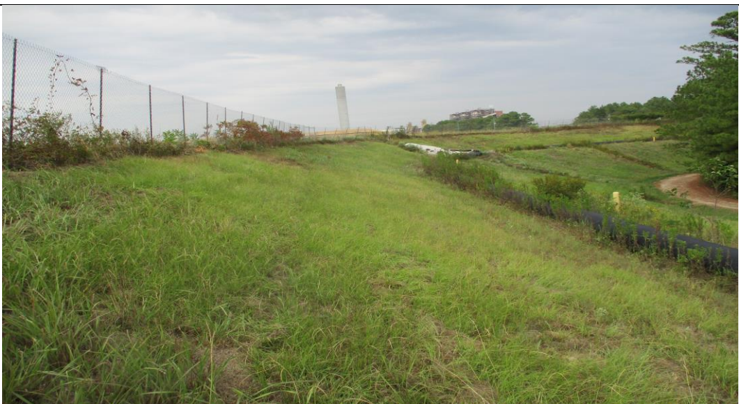
Photograph No. 4 Overall view of the east dike downstream slope.
