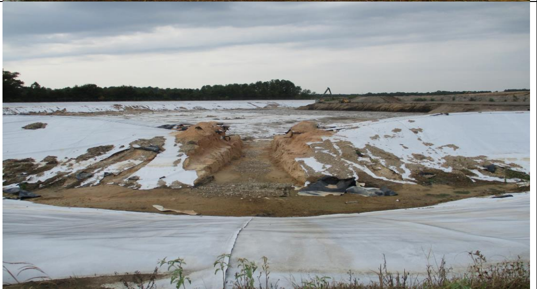
Photograph No. 14 Interior area service spillway removed.
