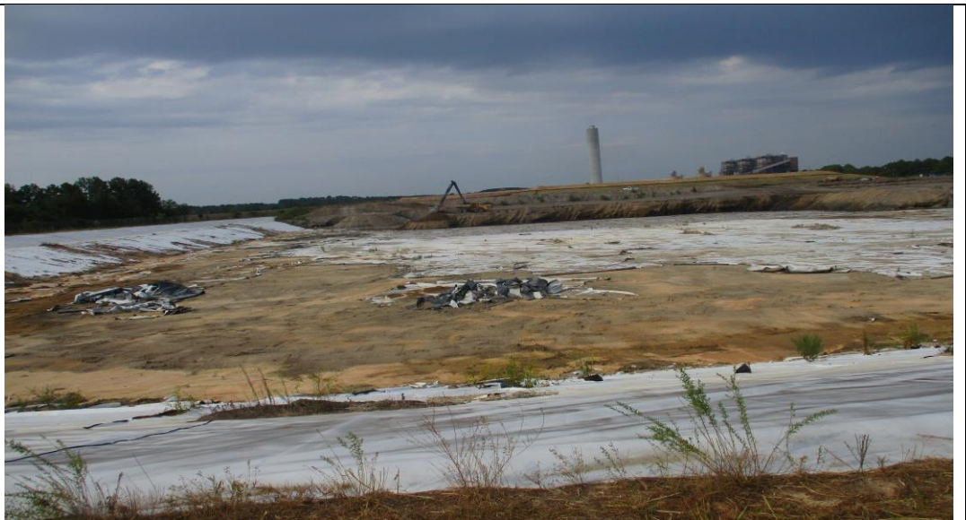
Photograph No. 13 Pond interior illustrating excavation of CCR materials.
