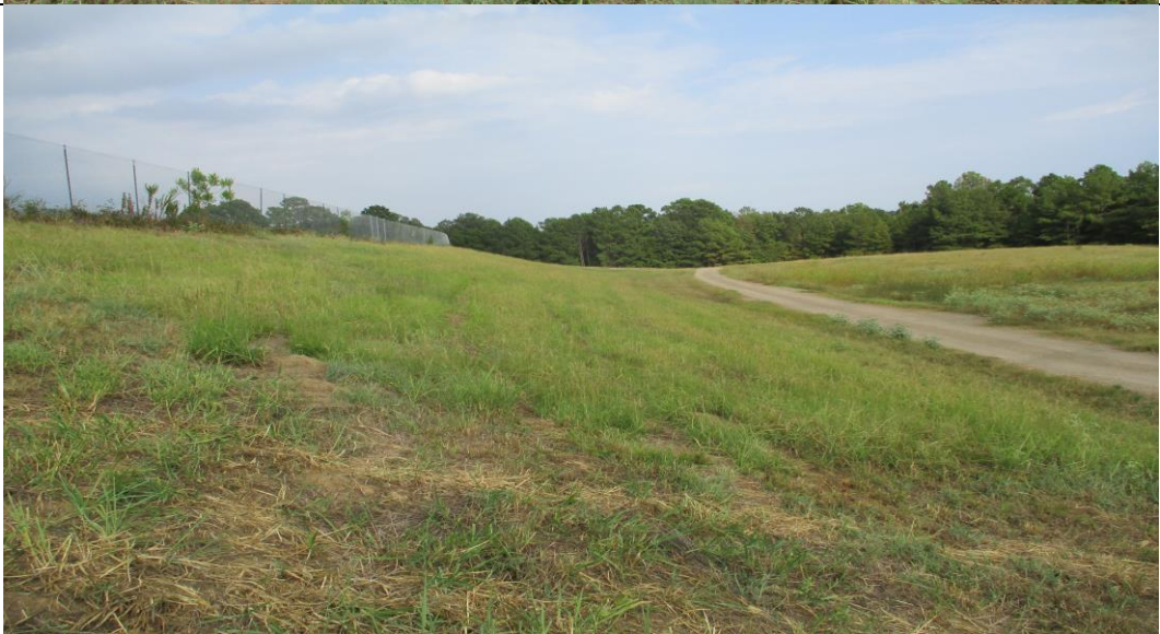
Photograph No. 6 Southeast downstream slope.
