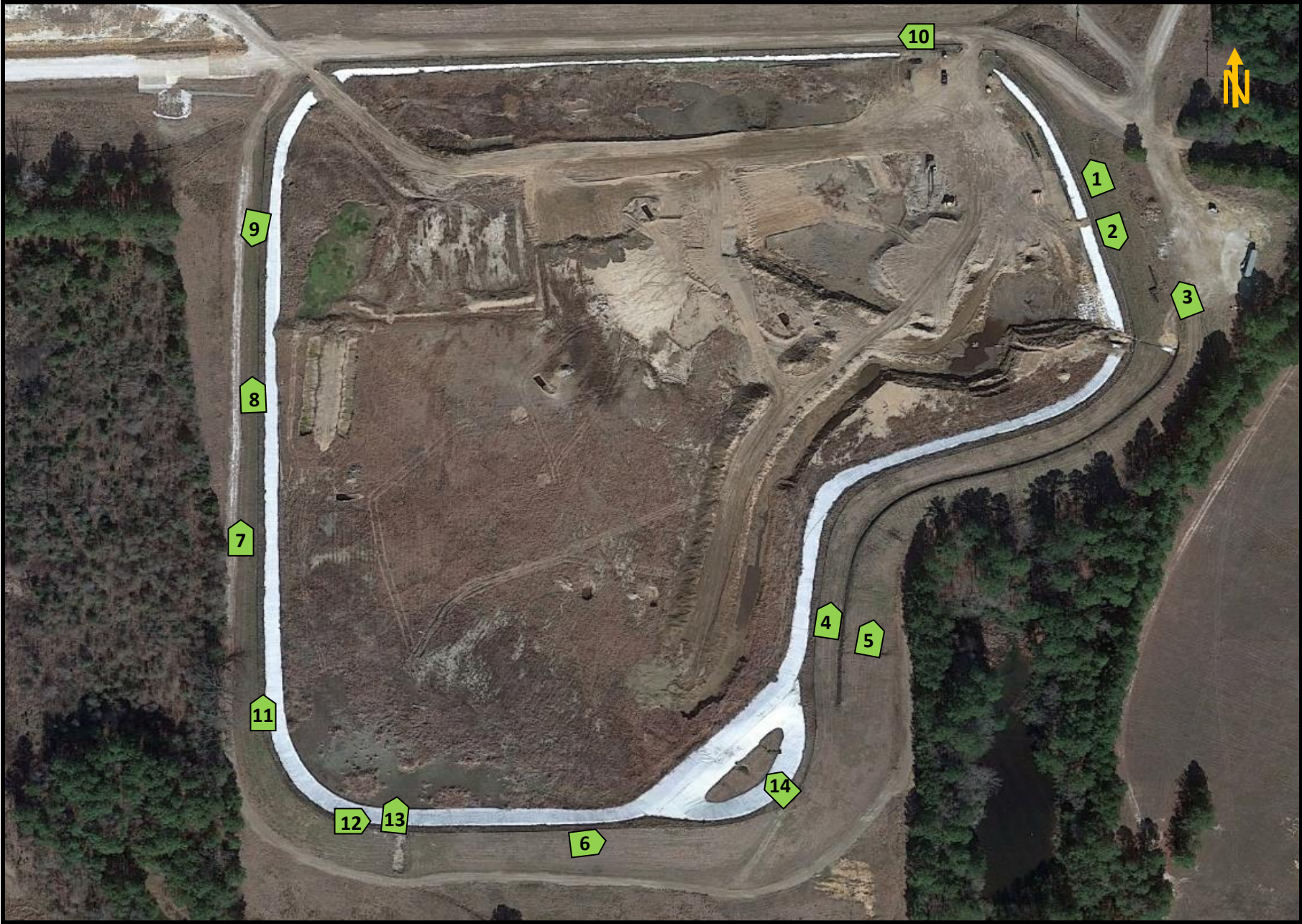
FIGURE 3 - PHOTOGRAPH LOCATION MAP BOTTOM ASH STORAGE POND, WELSH POWER PLANT, CASON, TX
