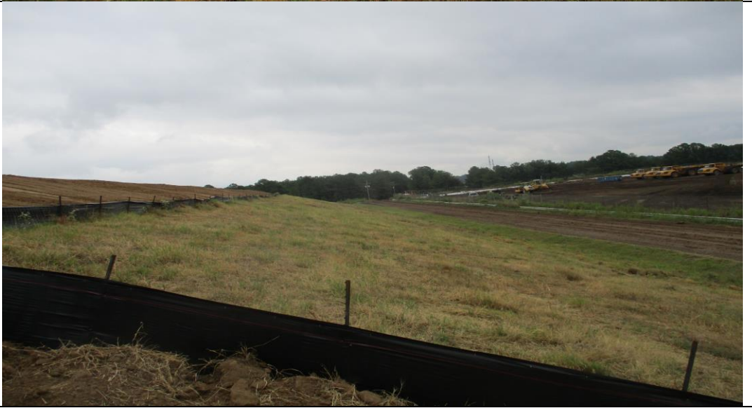
Photograph No. 17 South slope of the landfill (looking east).
