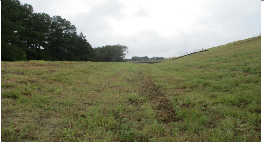
Photograph No. 1 View of the eastern slope (looking south).
