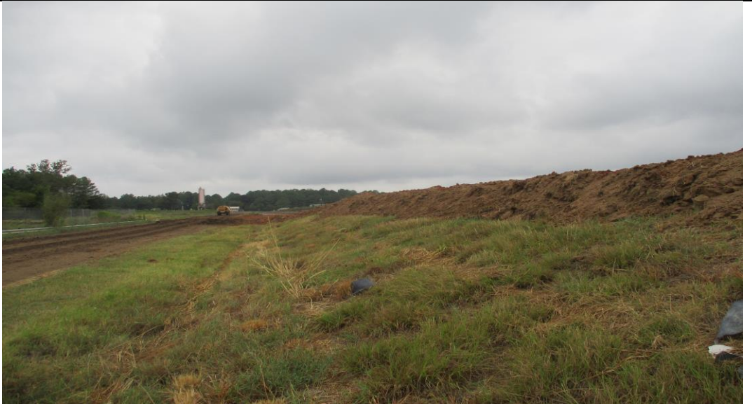
Photograph No. 16 South slope of the landfill (looking west).
