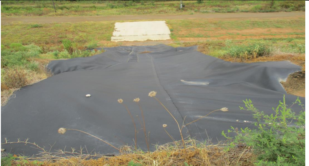
Photograph No. 7 View of the northern slope central let down channel.
