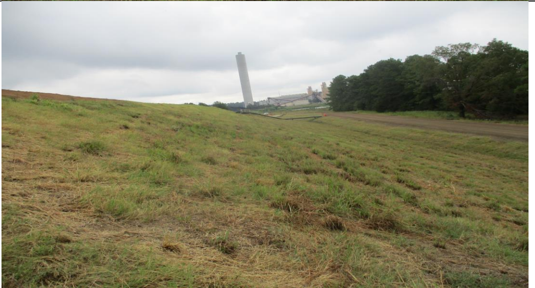
Photograph No. 2 View of the eastern slope (looking north).
