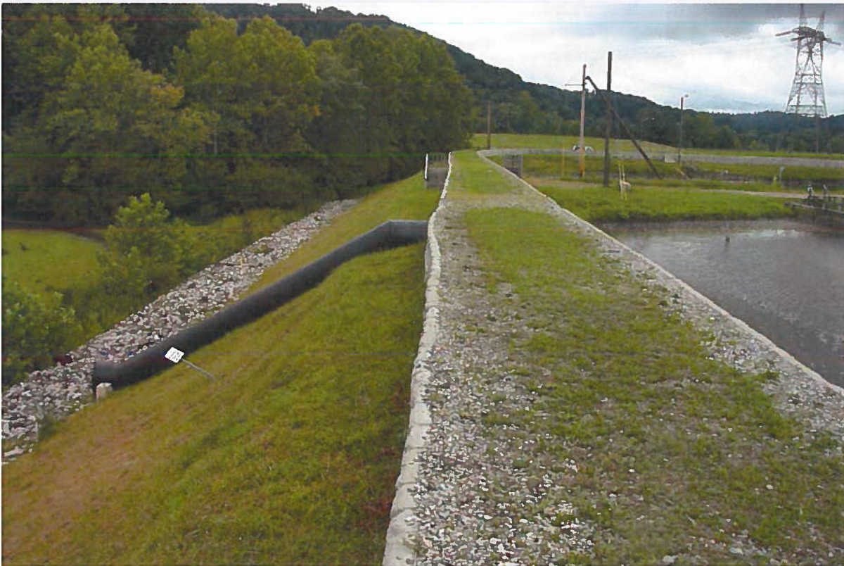
Photograph 2. Reclaim Pond Spillway Pipe and Downstream Slope.
