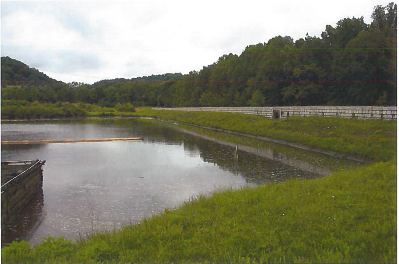
Photograph 6. Reclaim Pond and Upstream Slope.
