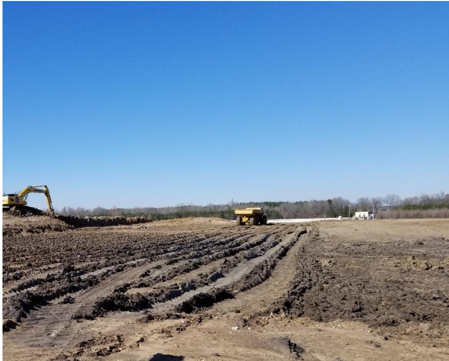
Looking north at proof-rolling subgrade.
