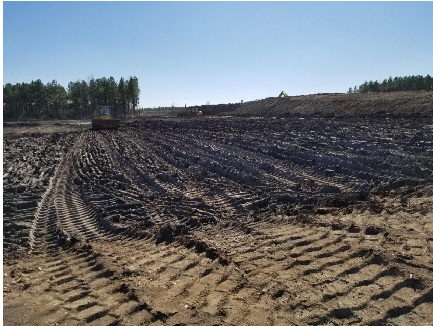
Looking south at sheep's foot compacting subgrade.
