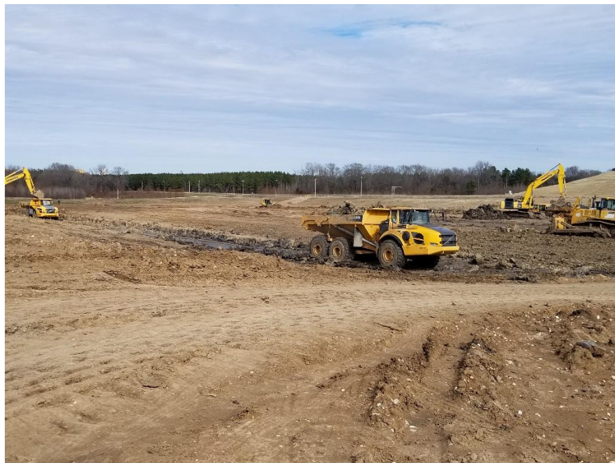
Haulers transporting structural fill material.
