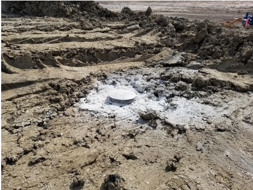
Bentonite placement over cap before concrete cover.
