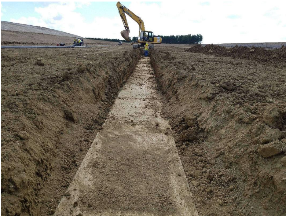
Looking south at excavator cutting protective cover for leachate lines.
