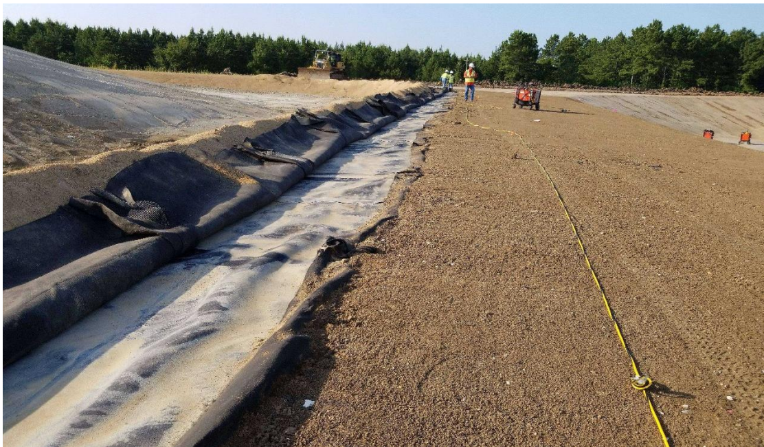
Looking south at exposing the geosynthetics tie in on the east berm.
