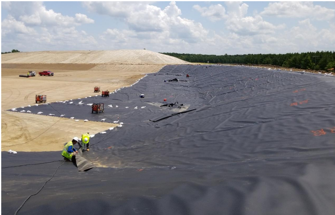
Looking east at deployed and seamed geomembrane on the south slope.
