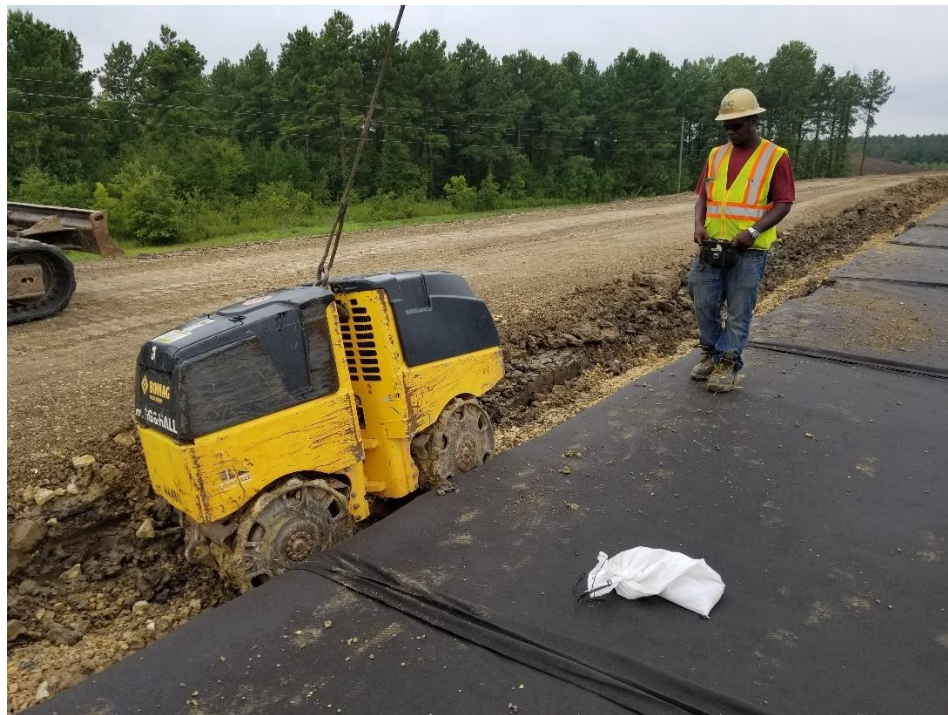
Compacting south geosynthetics anchor trench.
