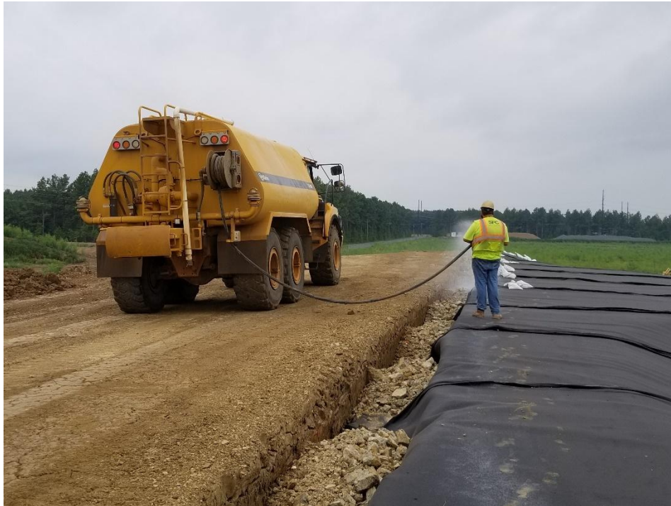
Looking west moisture conditioning anchor trench material prior to compaction.
