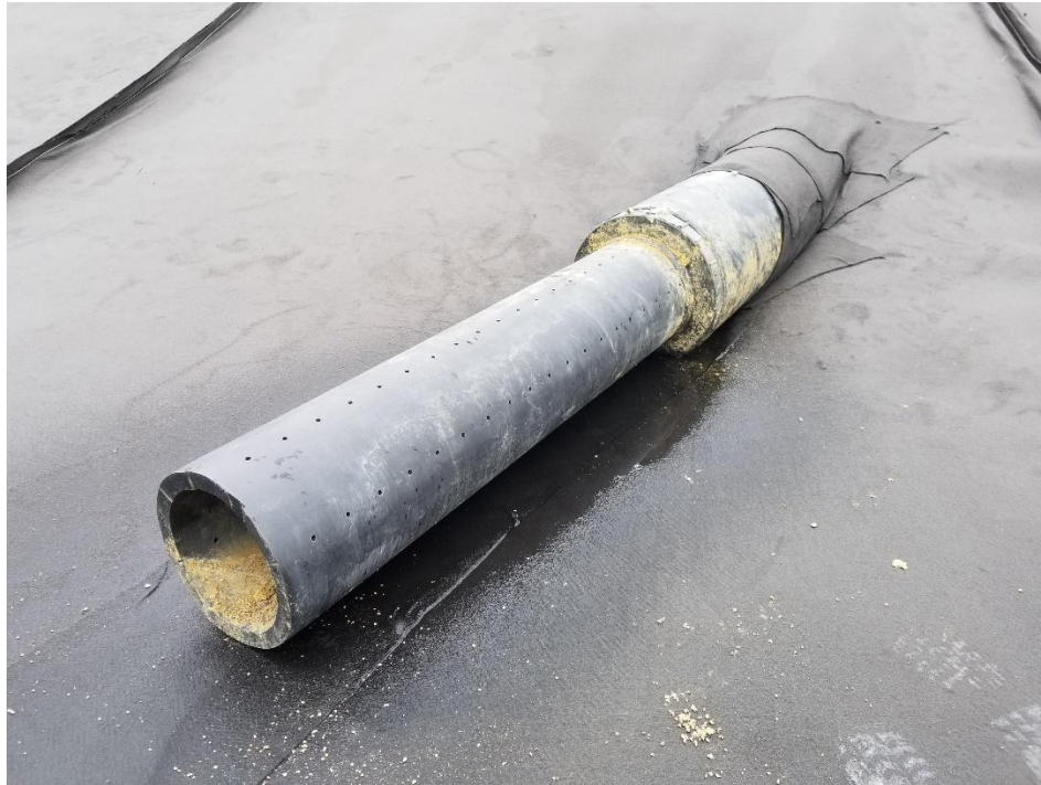
Looking at south leachate line penetration at south berm.
