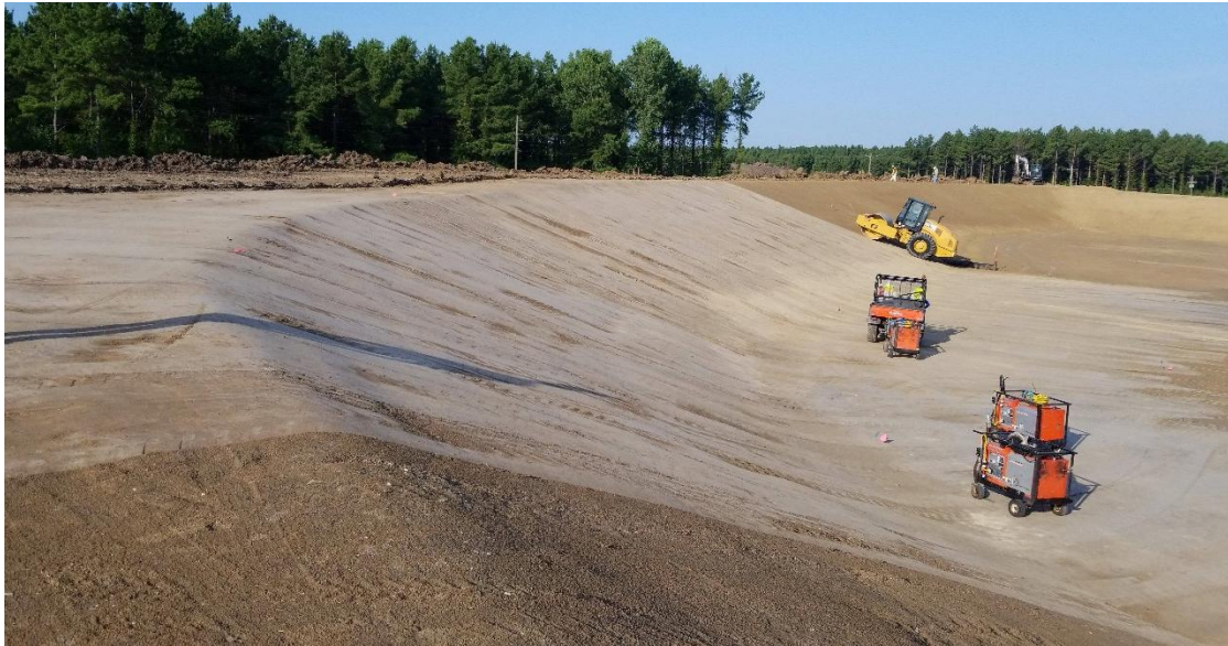
Looking southwest at smooth rolling subgrade in preparation for geomembrane deployment.
