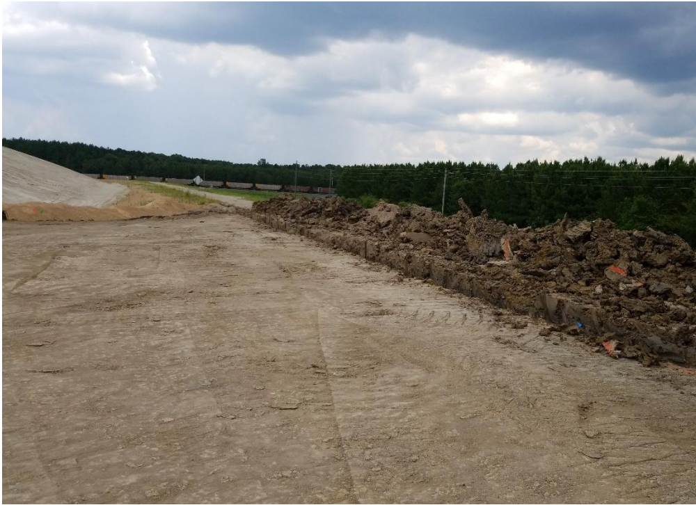
Looking east at cutting the south geosynthetics anchor trench.
