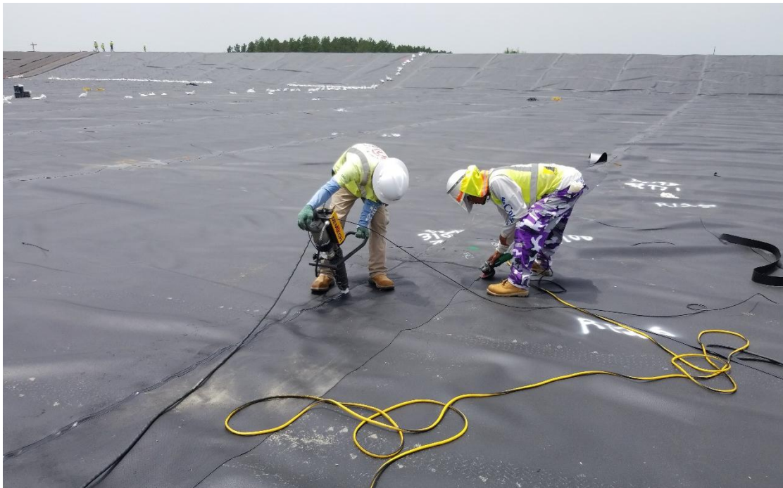
Looking at extrusion seaming preparation and welding geomembrane repair.
