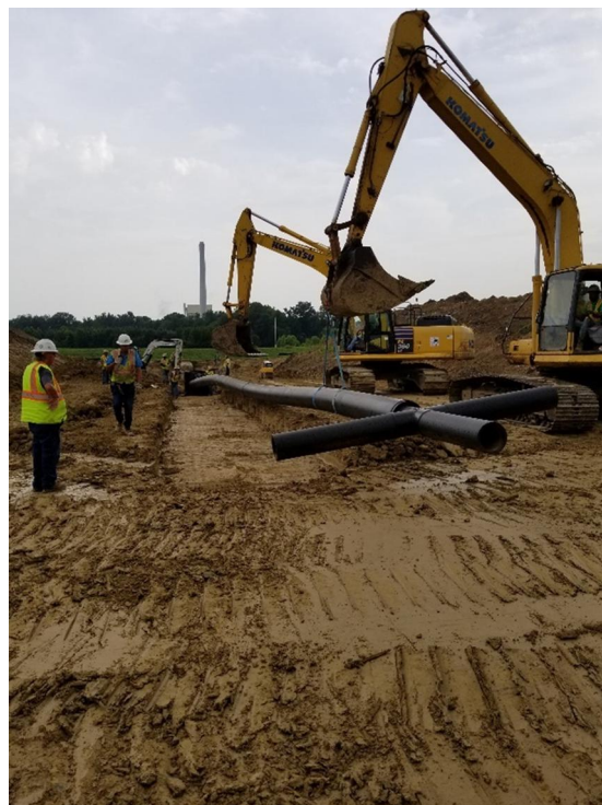
Looking north at excavators placing north leachate line in north berm.
