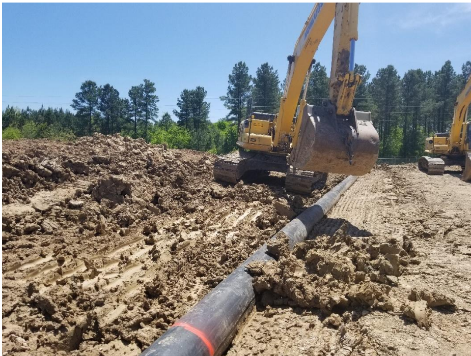
Looking south at placement of the south leachate line.
