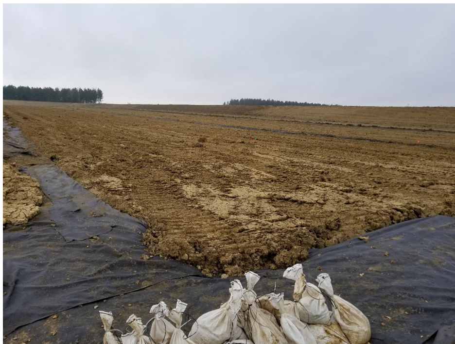
Looking southwest at leachate lines and gravel covered by geotextile.
