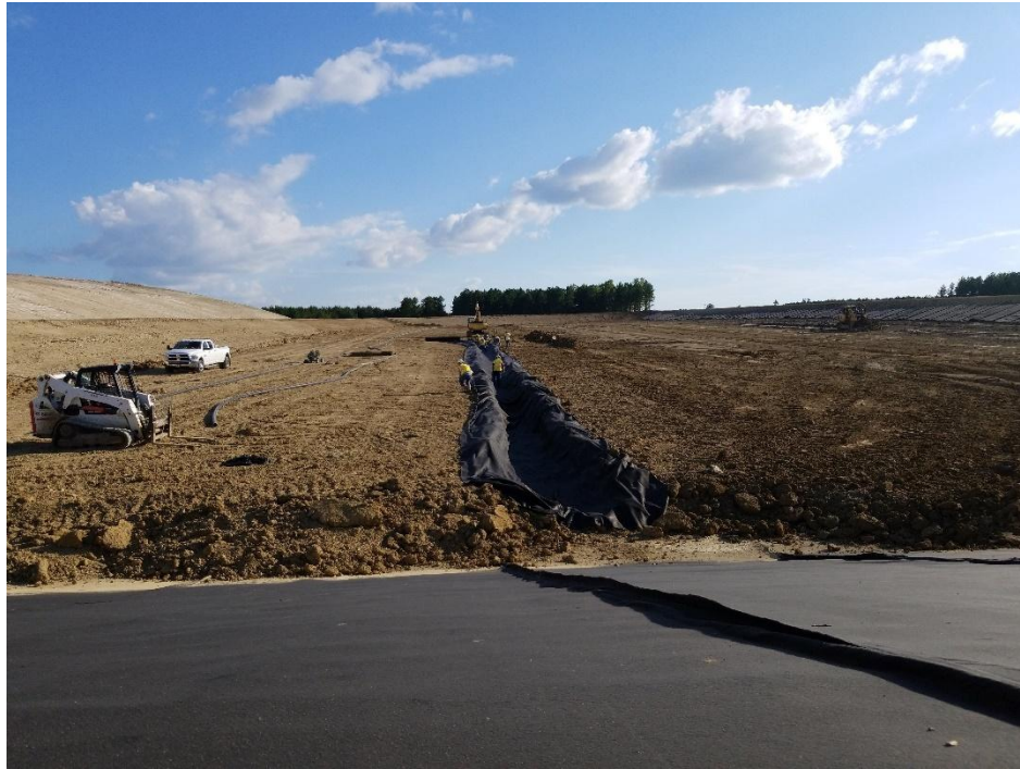
Looking south at placement of geotextile in leachate trench.
