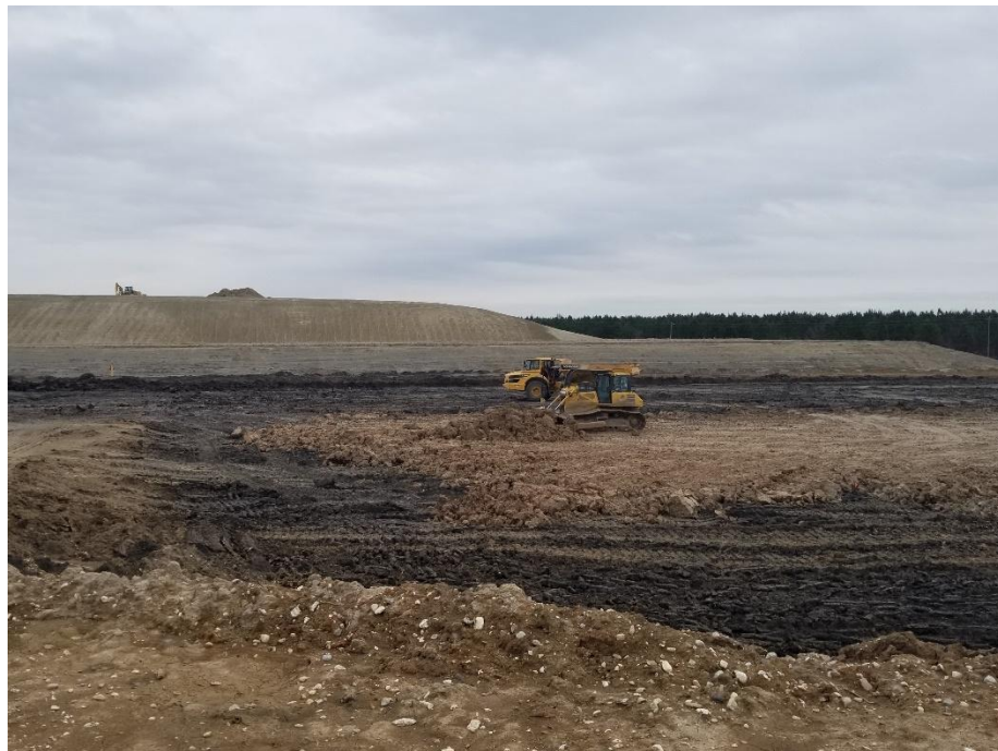
Looking east at dozer spreading subgrade material to bring to elevation.
