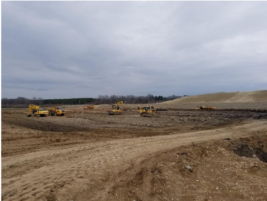
Looking northeast at hauling operation of subgrade.
