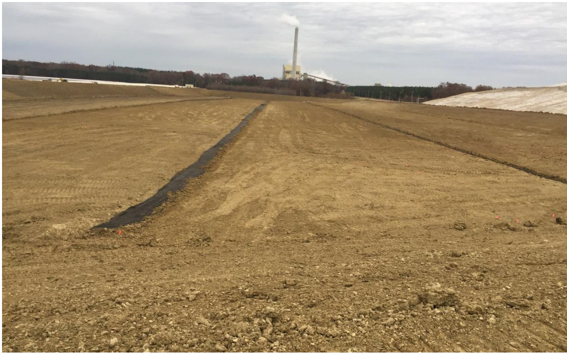
Looking north at completed protective cover layer.
