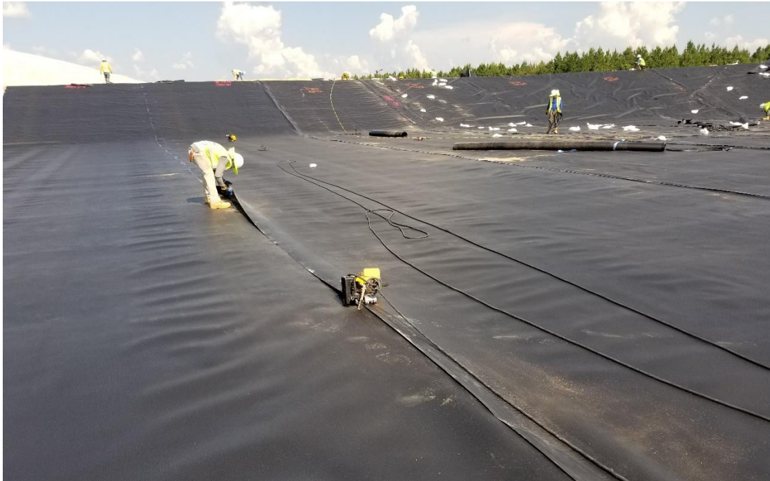
Looking east at cleaning and fusion welding geomembrane seam.
