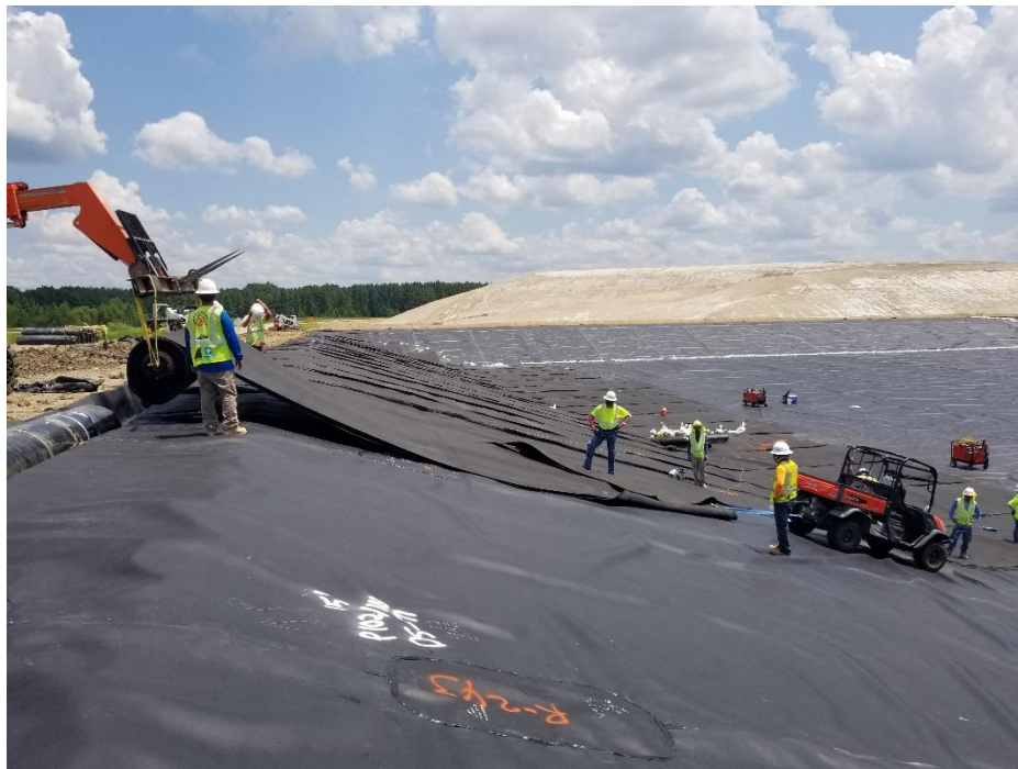
Looking east at ESI deploying geocomposite on north berm.
