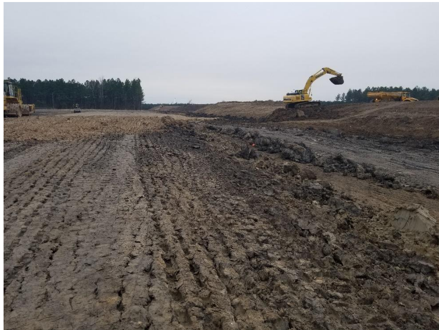
Looking south at Excavator cutting overburden and loading into hauler.
