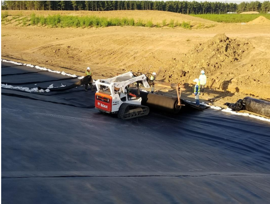
Looking southwest at deployment of geocomposite on west slope.
