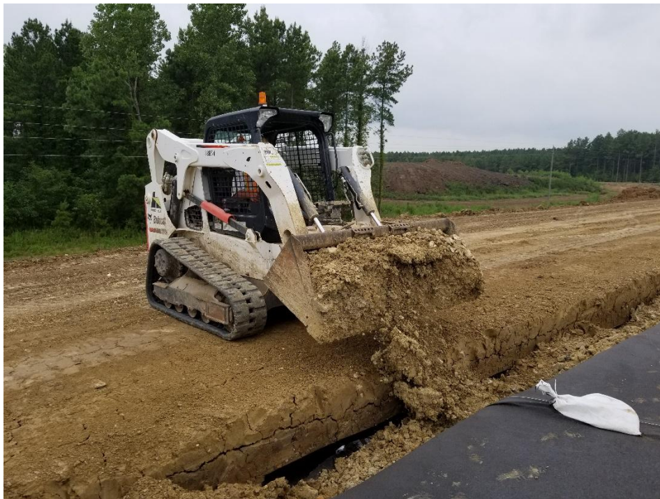
Looking southwest at skidsteer backfilling south geosynthetics anchor trench
