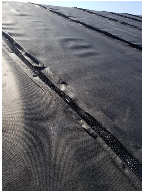
Zip-ties used to connect geonet between geocomposite panels.
