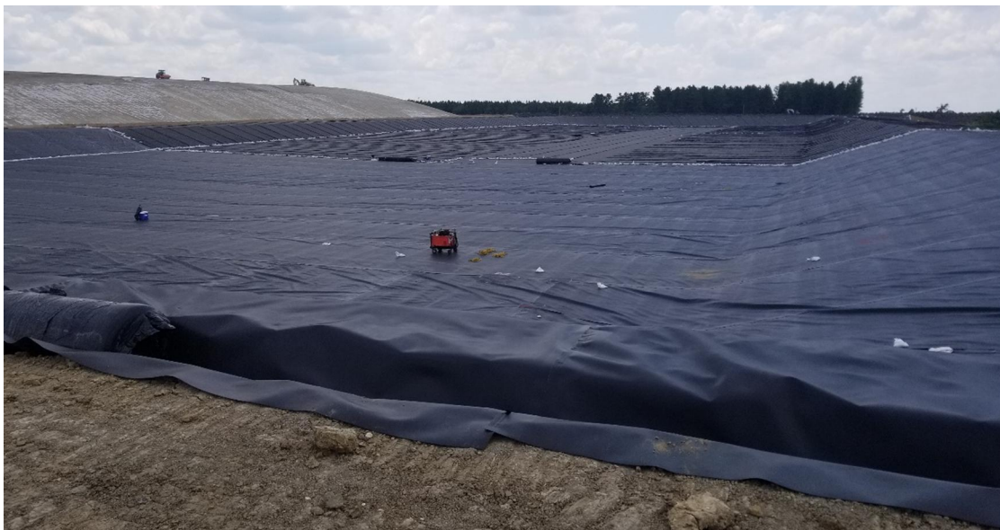
Looking south at completed geomembrane deployment and partial deployment of geocomposite.
