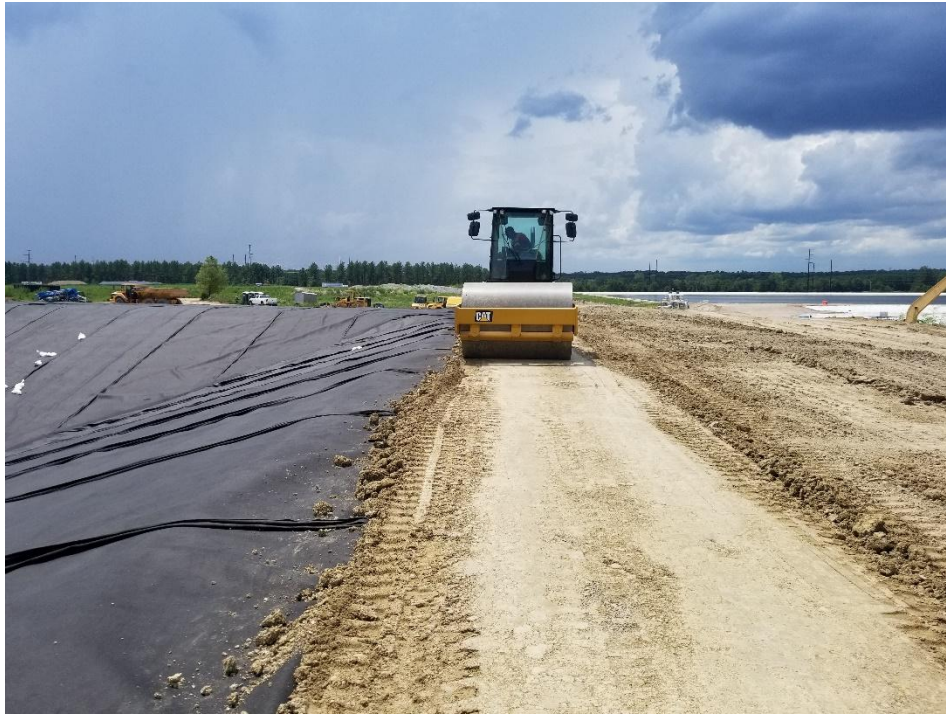
Looking west at drum compacting north geosynthetics anchor trench.
