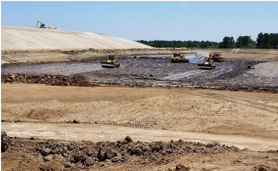
Looking southeast at grading, moisture conditioning and compacting clay liner.
