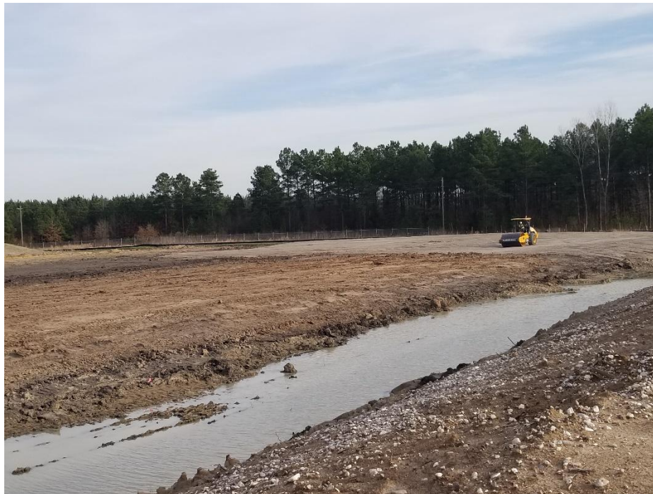
Looking southeast at smooth drum sealing west berm before expected rain.
