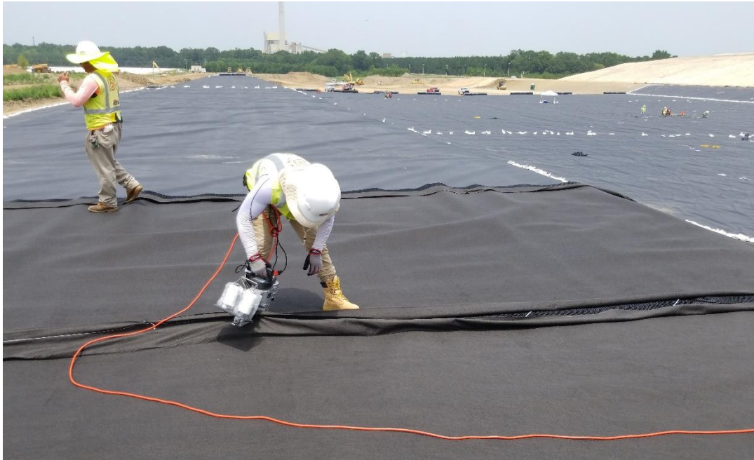
Looking at sewing the geotextile layer of the geocomposite.
