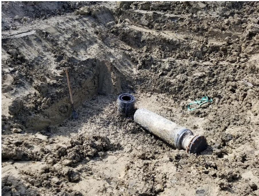
Pipe after cutting cleanout to reduce top elevation.
