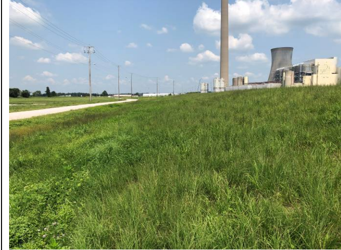
Photograph 1: #W View of the embankment dike of the west bottom ash pond, looking north.
