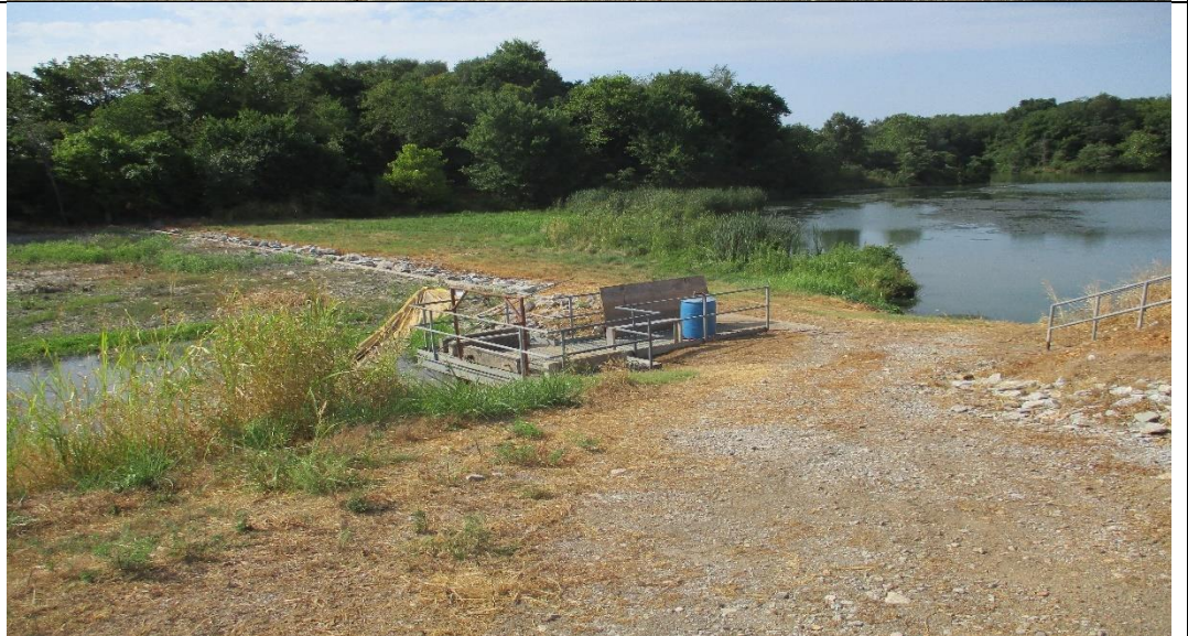
PHOTO #12 Overflow discharge structure.
