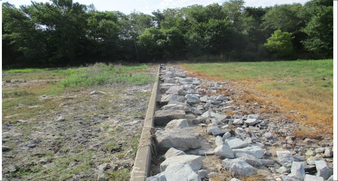
PHOTO #10 Emergency spillway concrete sill (looking south).
