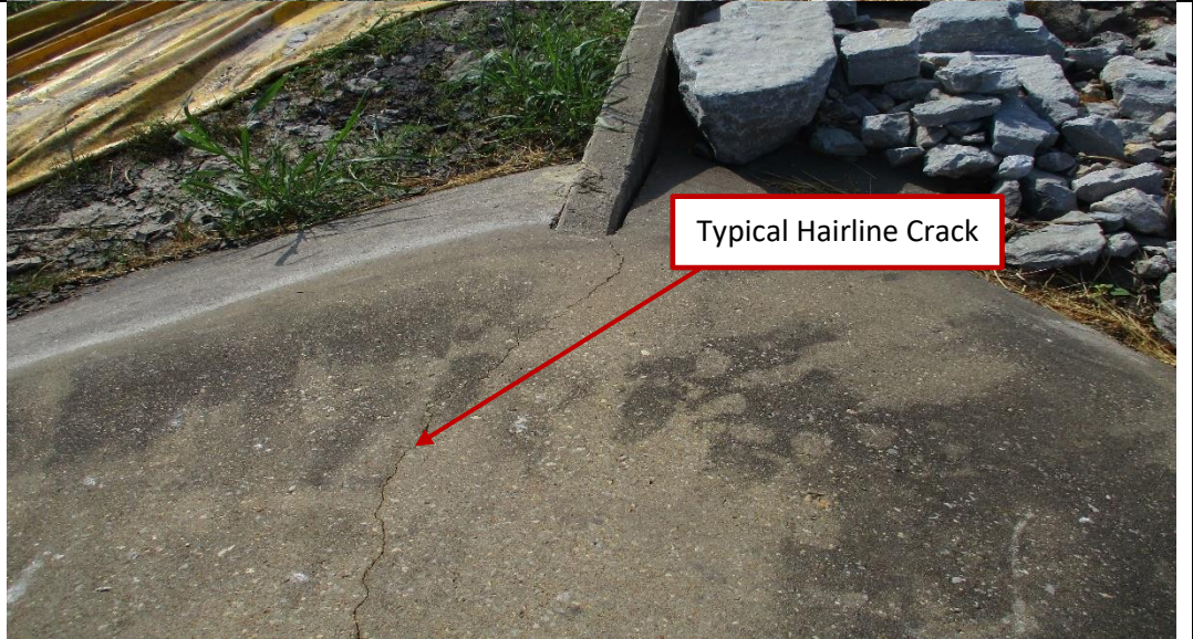
PHOTO #11 Upstream north slope (looking west).
