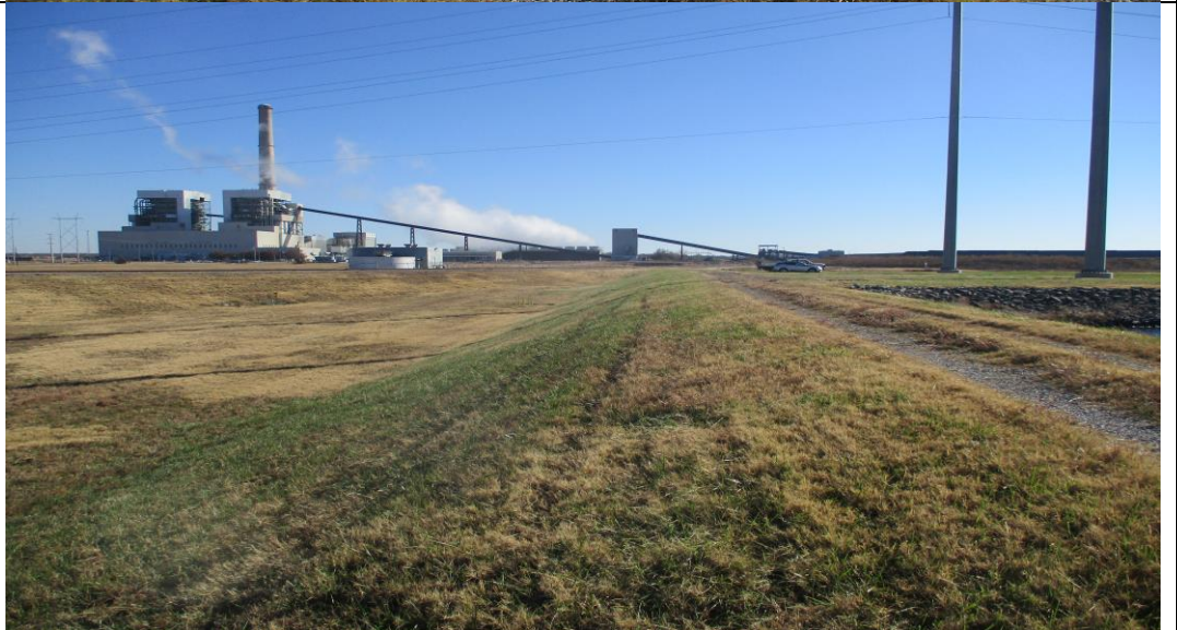
Photograph No. 5 Downstream slope of the northwest dike section.
