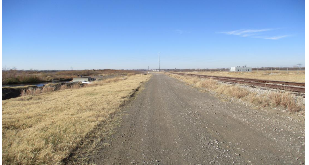
Photograph No. 17 North dike crest (looking west).
