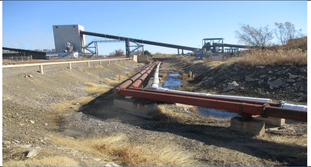
Photograph No. 16 Sluice pipes support.
