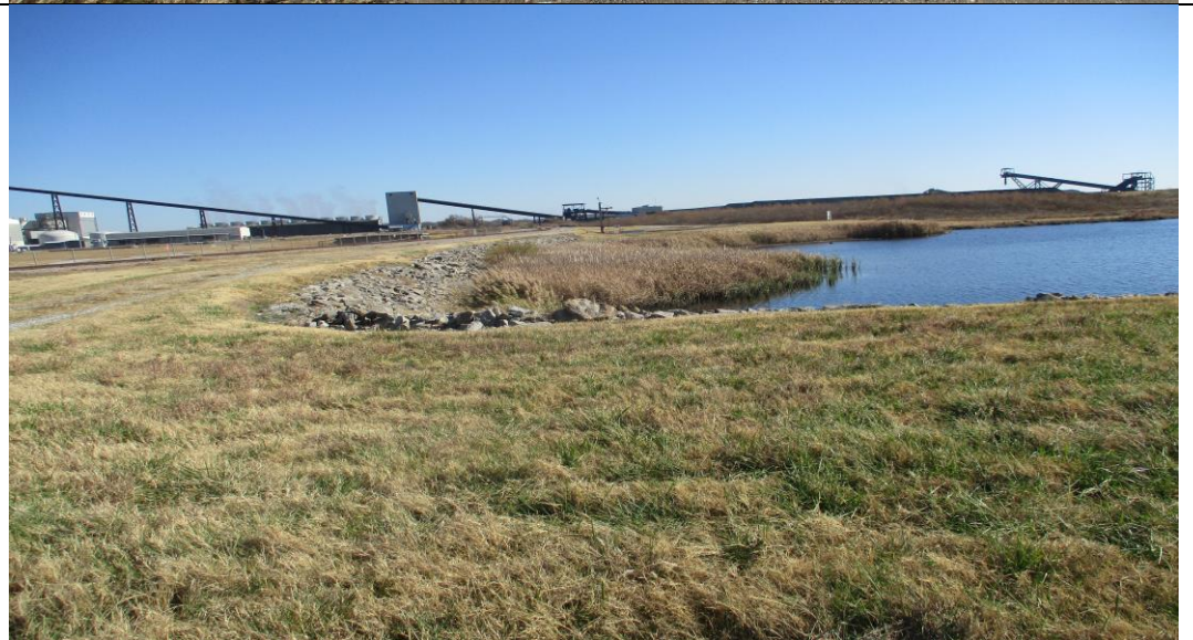
Photograph No. 18 Upstream slope of the northeast dike section.
