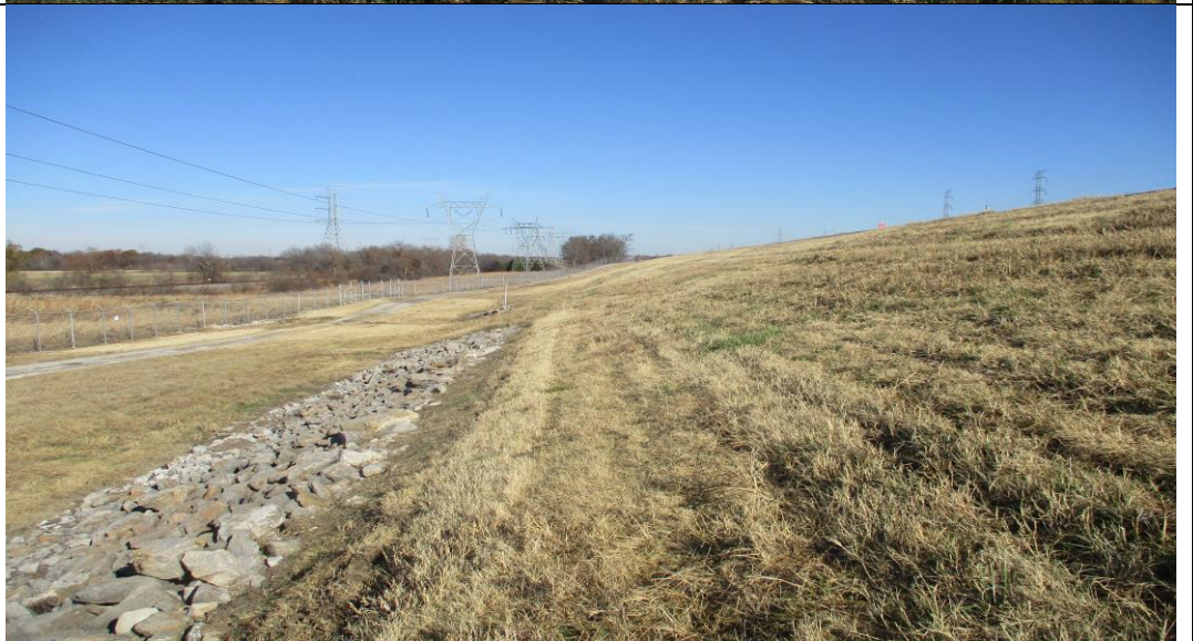
Photograph No. 6 Downstream slope toe drain (looking north).
