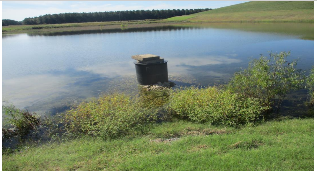
Photograph No. 19 Overflow discharge pipe.
