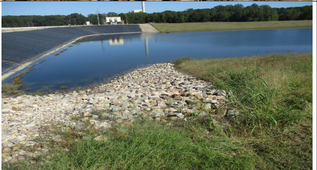
Photograph No. 24 West interior slope.
