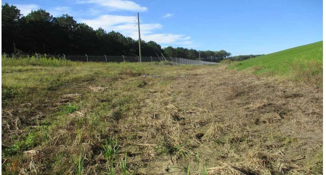
Photograph No. 7 Toe ditch (looking west).
