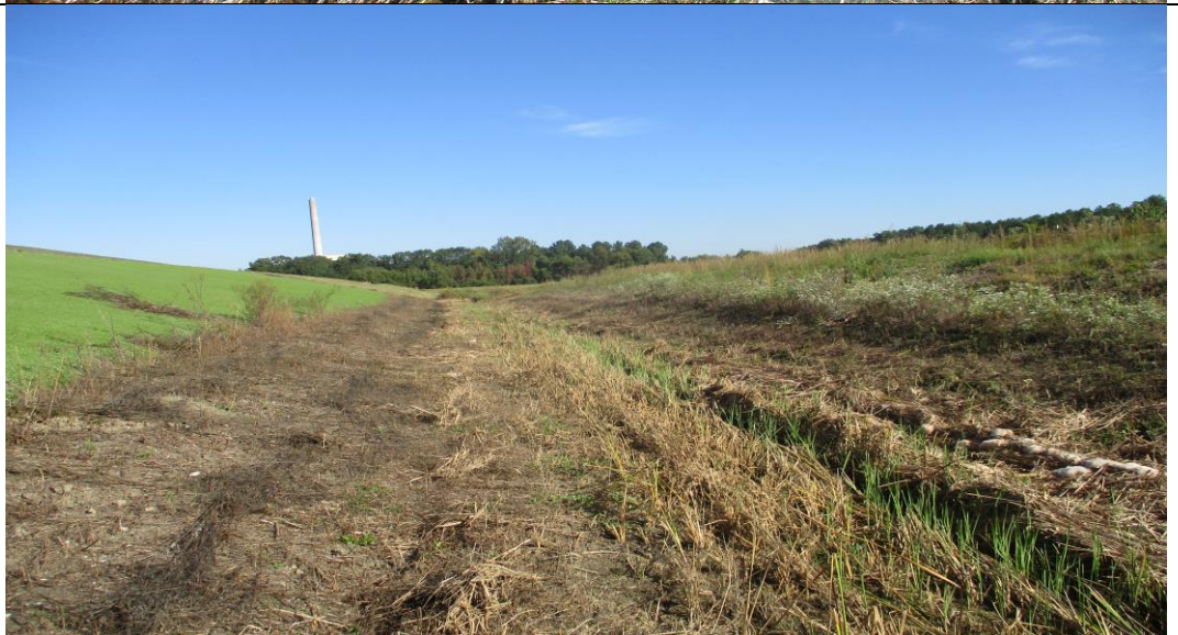
Photograph No. 9 Toe ditch east side (looking north).
