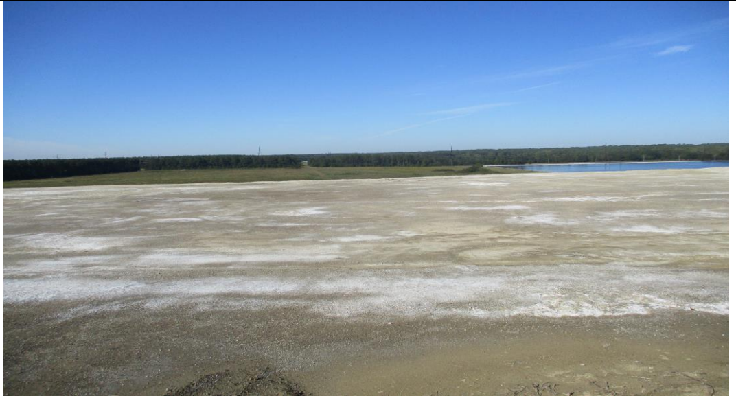
Photograph No. 4 Top of Cell 1.
