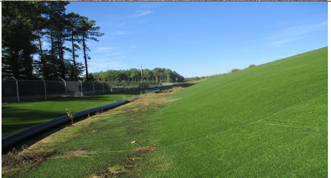
Photograph No. 6 Landfill support berm and storm water ditch (looking west).
