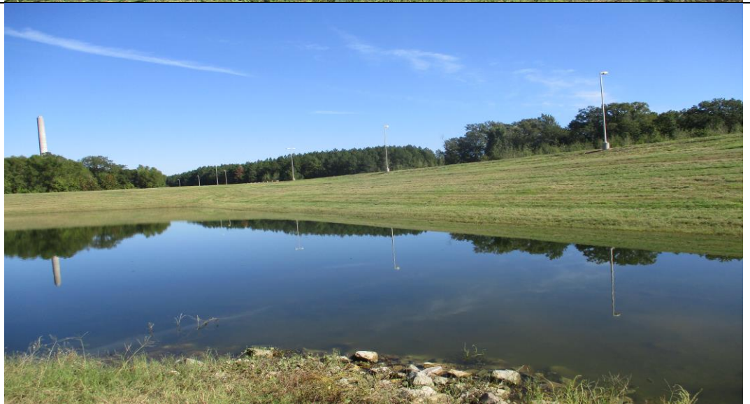
Photograph No. 21 Typical condition of the leachate pond interior.
