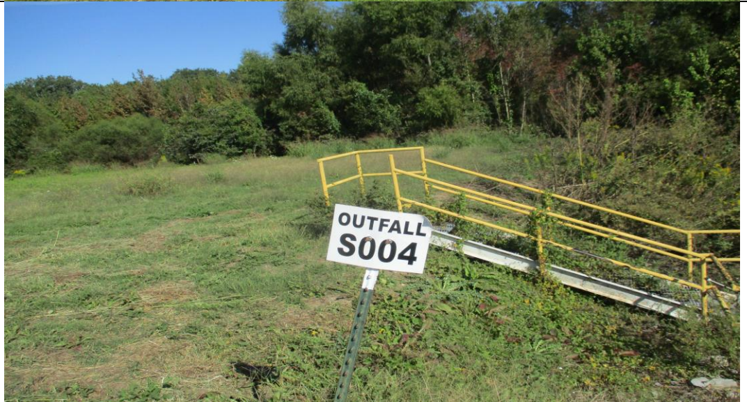
Photograph No. 20 Overflow discharge structure.
