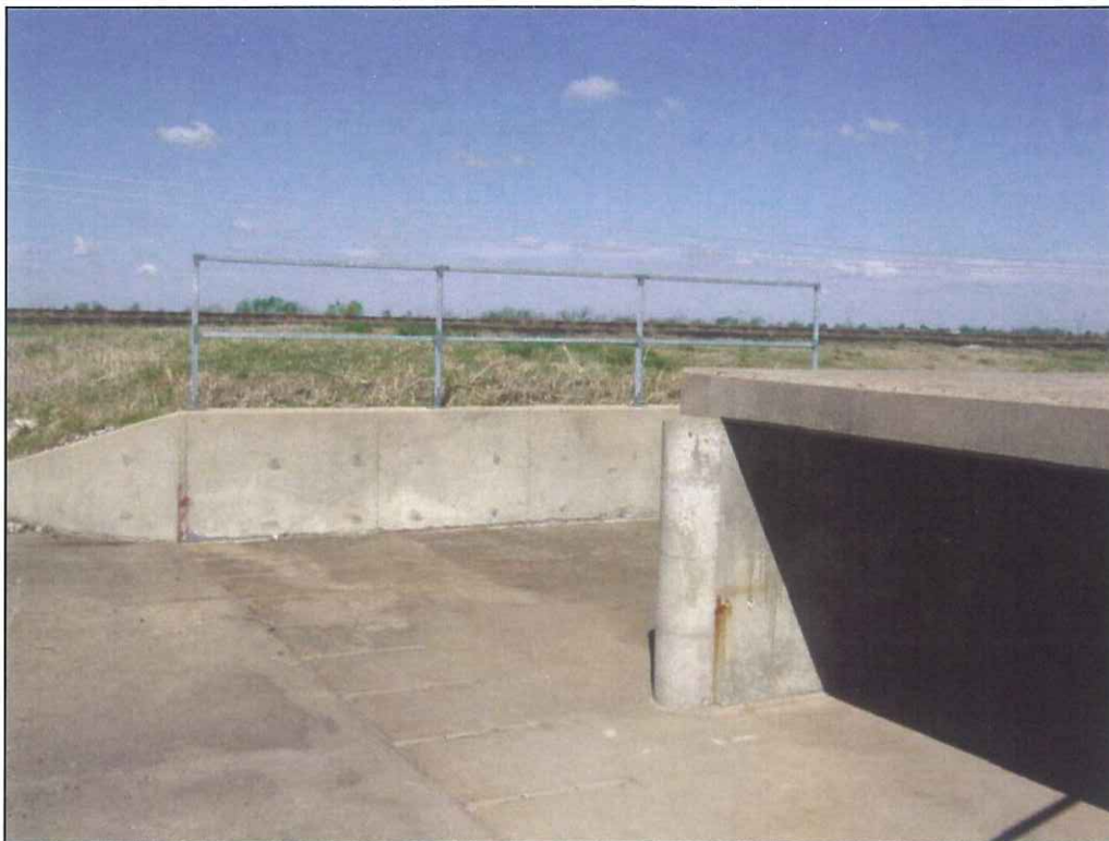
Figure 5 – Bottom Ash Pond Spillway
