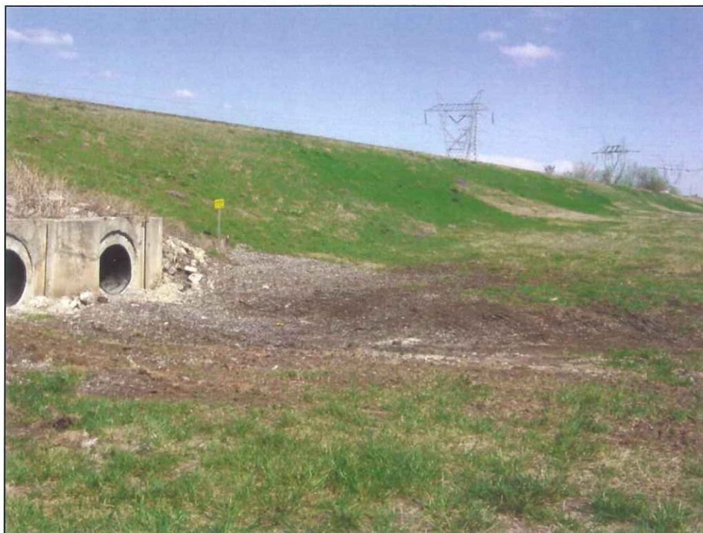
Figure 6 – Downstream Basin with Culverts
