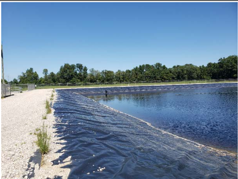
Photo # 7 North Leachate pond (exposed liner portion).
