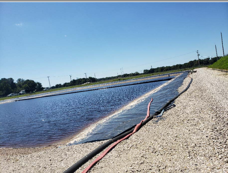
Photo # 8 West Leachate pond – West pond exposed liner portion.
