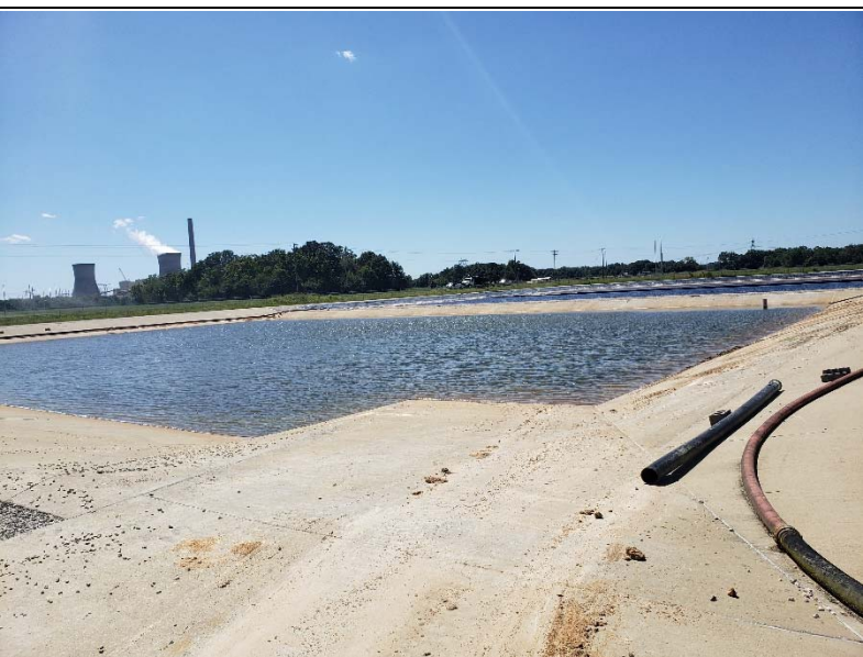
Photo # 9 West Leachate pond (concrete lined portion) – Concrete exposed portion being used to remove mineral precipitation from sulfate reduction.
