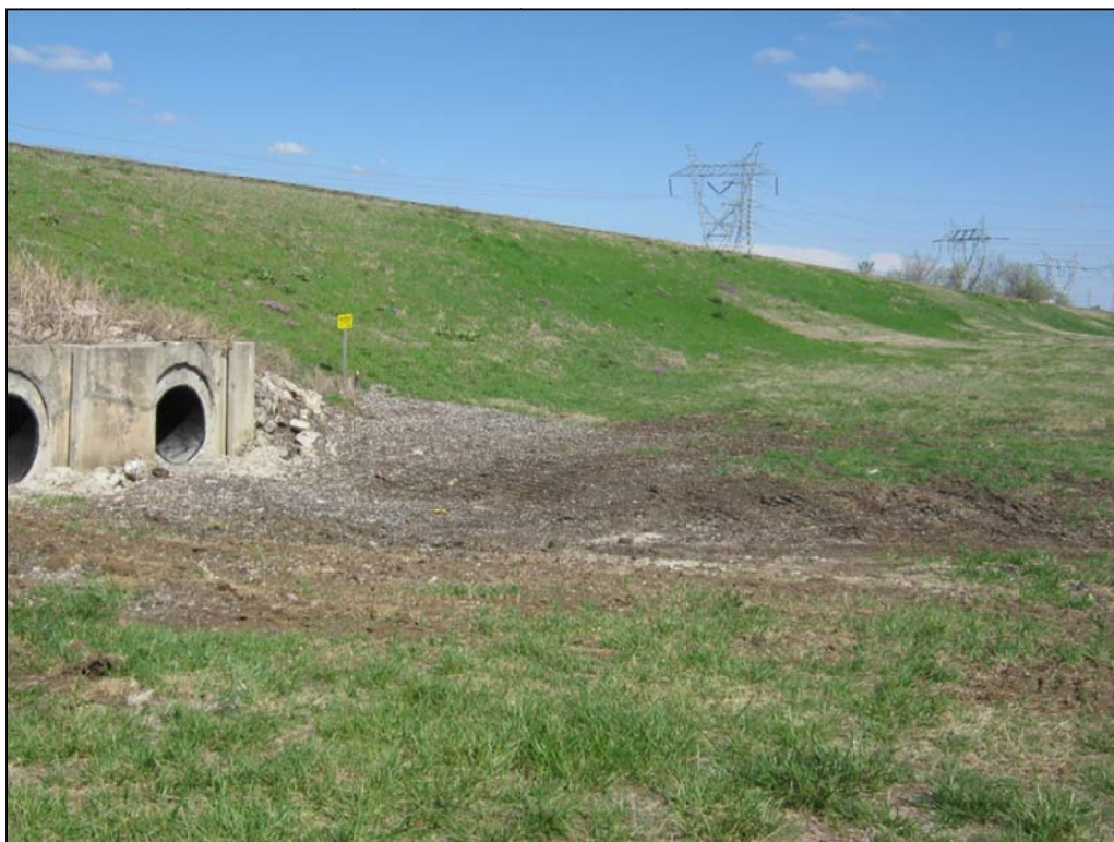
Figure 6 – Downstream Basin with Culverts
