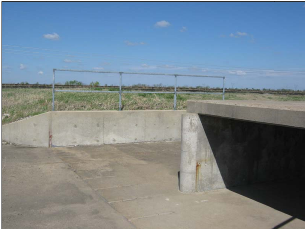
Figure 5 – Bottom Ash Pond Spillway
