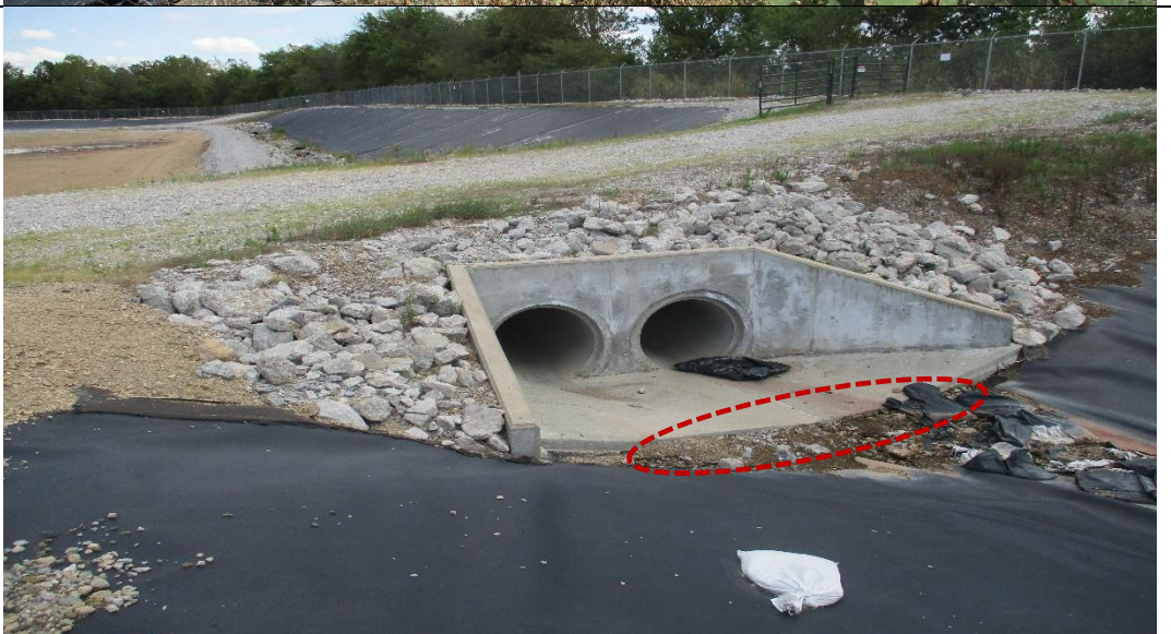
Photograph No. 12 South side perimeter runoff ditch and pipe culvert inlet.
