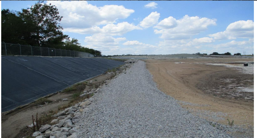
Photograph No. 18 Contact water ditch.
