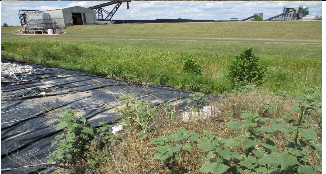
Photograph No. 11 Cell 1 area runoff perimeter water ditch (looking northwest).
