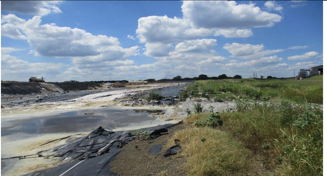
Photograph No. 10 Cell 1 surface graded (looking west).
