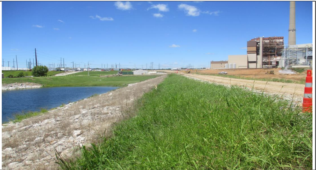
Photograph No. 7 Downstream slope (looking north).
