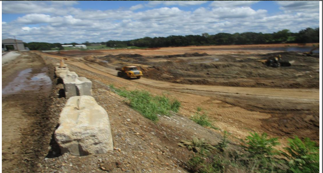
Photograph No. 9 The north embankment (looking east).
