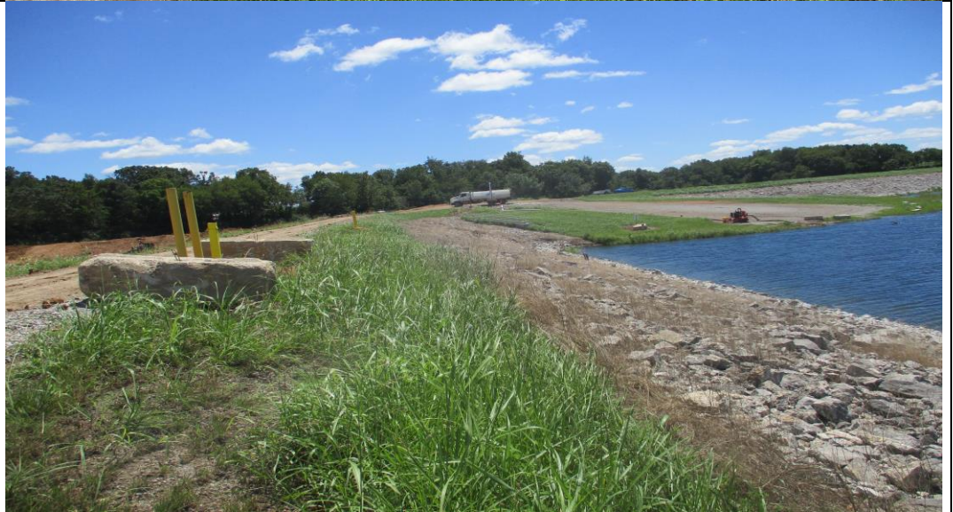
Photograph No. 8 Downstream slope (looking south).
