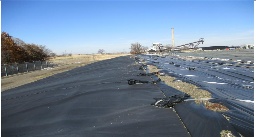
Photograph No. 1 Cell 4 berm and access road (looking north).
