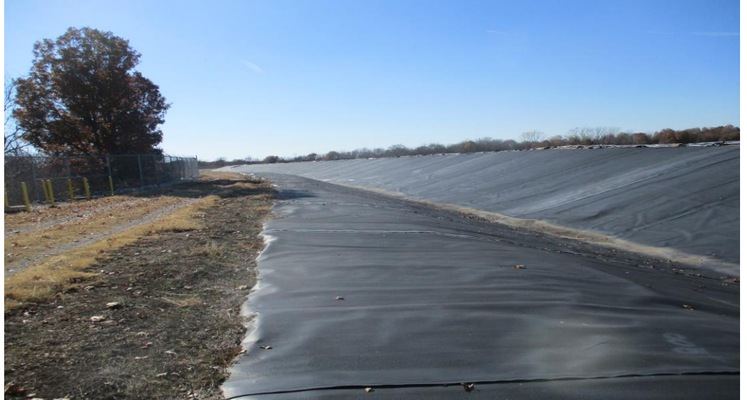
Photograph No. 10 Cell 2 access road and perimeter berm.
