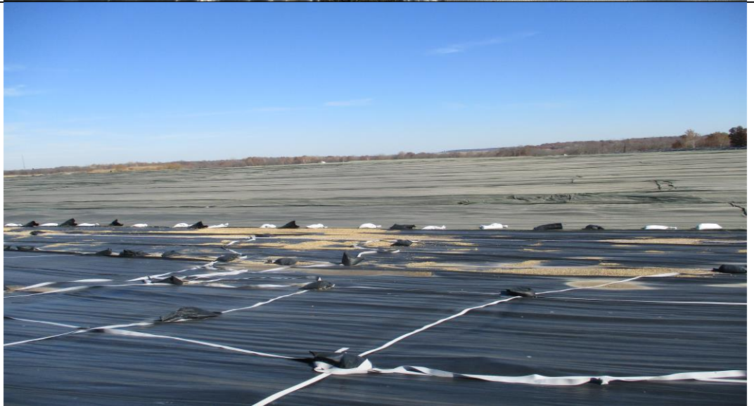
Photograph No. 3 Overall view of Cell 4.
