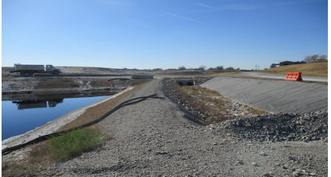
Photograph No. 16 North side ditch adjacent to the leachate pond.
