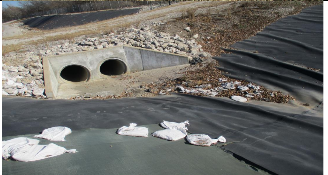
Photograph No. 14 South perimeter ditch pipe culvert inlet.
