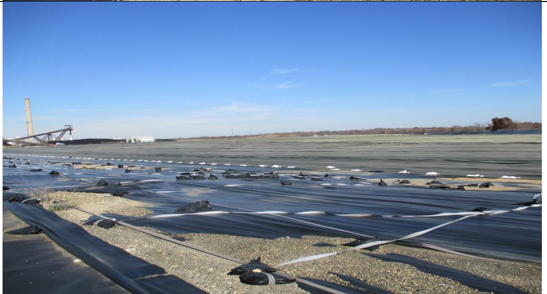
Photograph No. 6 Overall view of Cell 3 with rainflap and wind defender.
