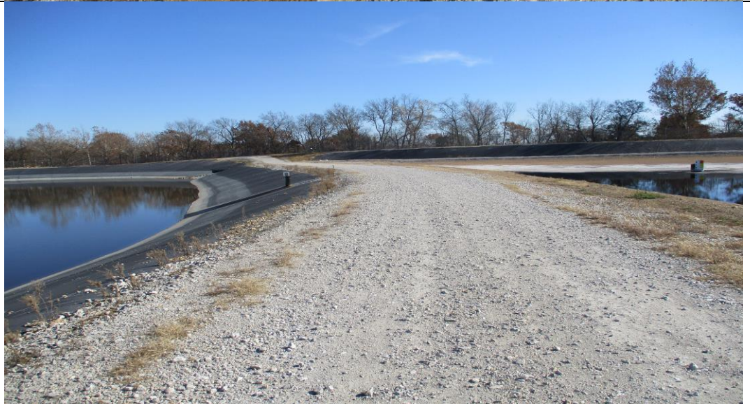
Photograph No. 23 Dike between the Basin C and the leachate pond
