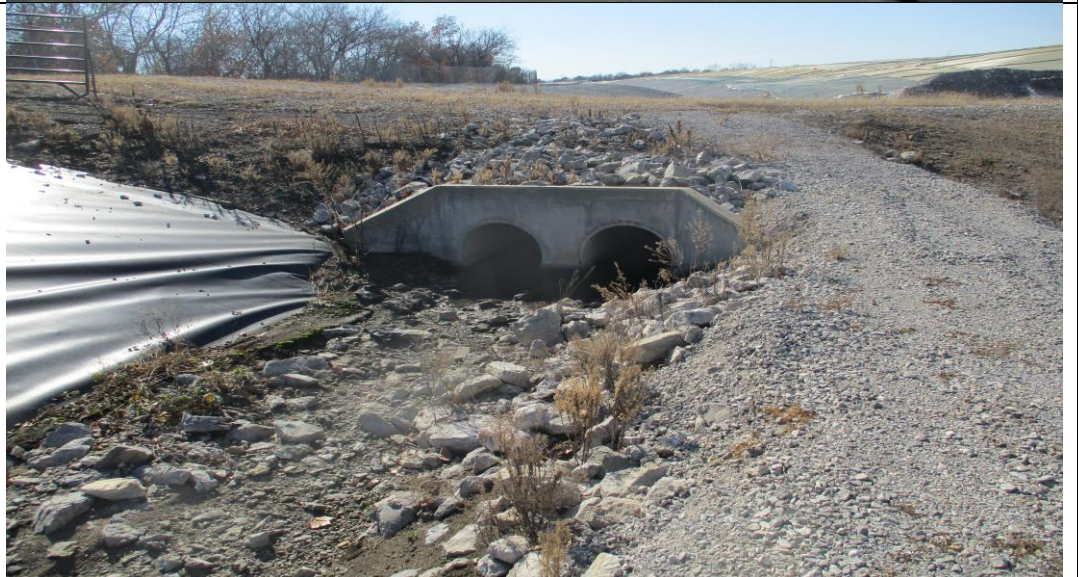
Photograph No. 15 South perimeter ditch pipe culvert outlet.
