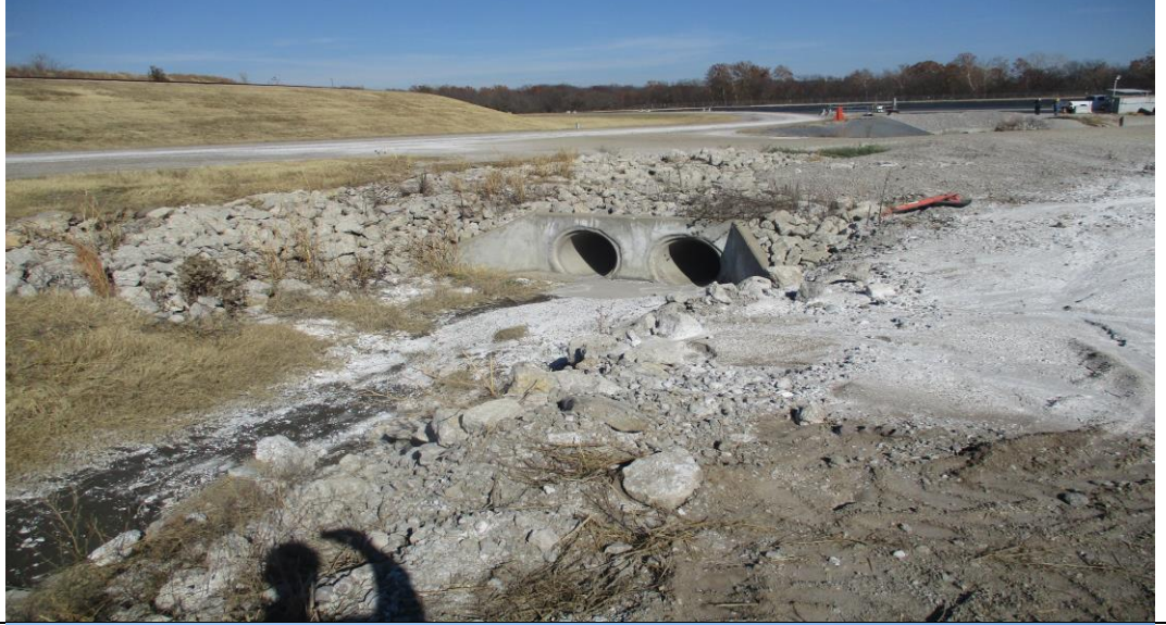
Photograph No. 17 North side ditch adjacent to Cell 1.
