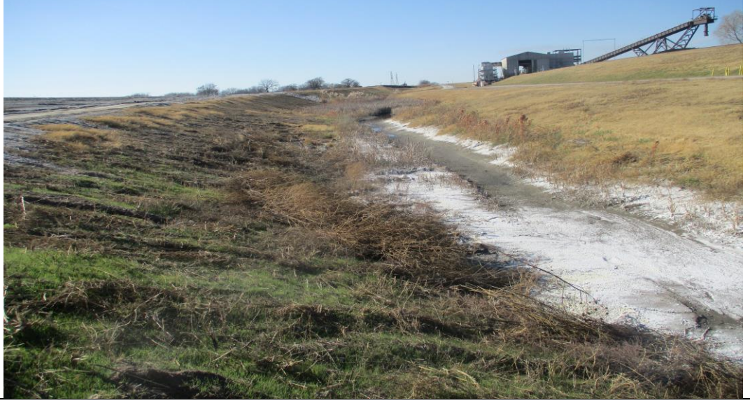
Photograph No. 18 North ditch (looking west).
