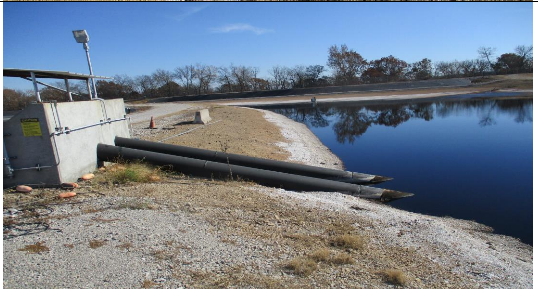
Photograph No. 21 Interior slope of the east dike.
