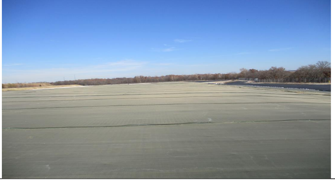
Photograph No. 9 Cell 2 area with rainflap and wind defender.
