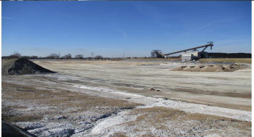
Photograph No. 11 Overall view of Cell 1.
