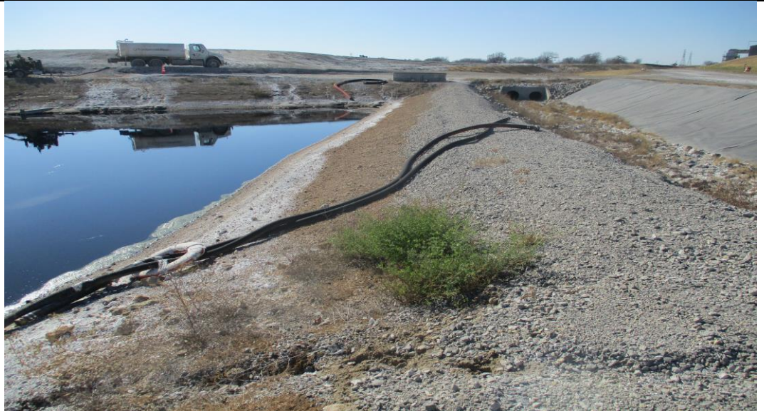
Photograph No. 22 North dike of the leachate pond.
