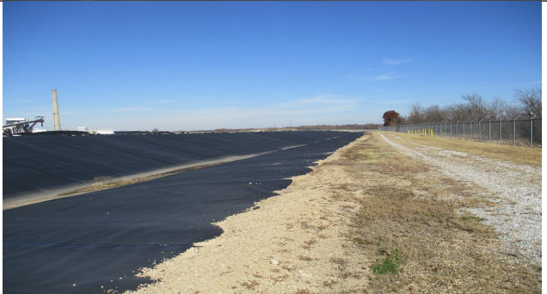
Photograph No. 5 Cell 3 perimeter berm and access road (looking northeast).
