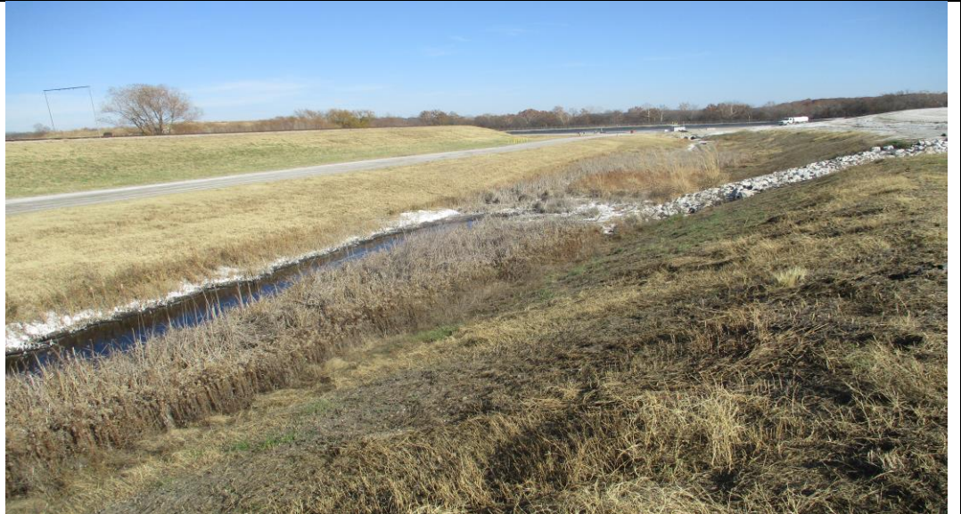
Photograph No. 13 Contact water ditch.
