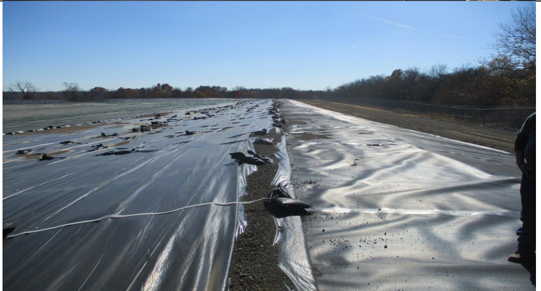
Photograph No. 2 Cell 4 and berm (looking south).
