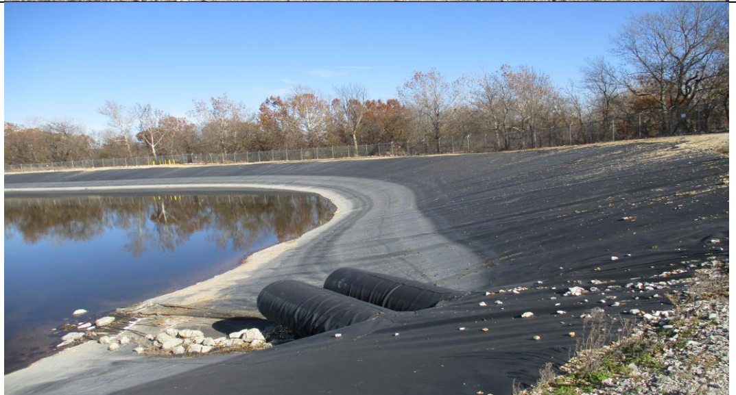
Photograph No. 24 Interior slope of Basin C.
