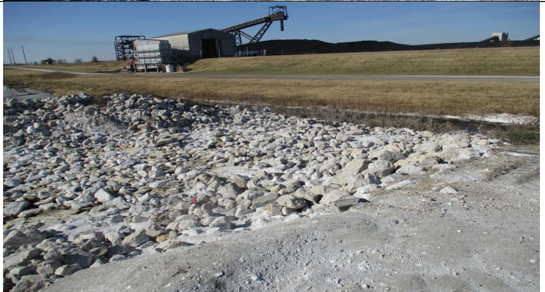
Photograph No. 12 Contact water channel of Cell 1.
