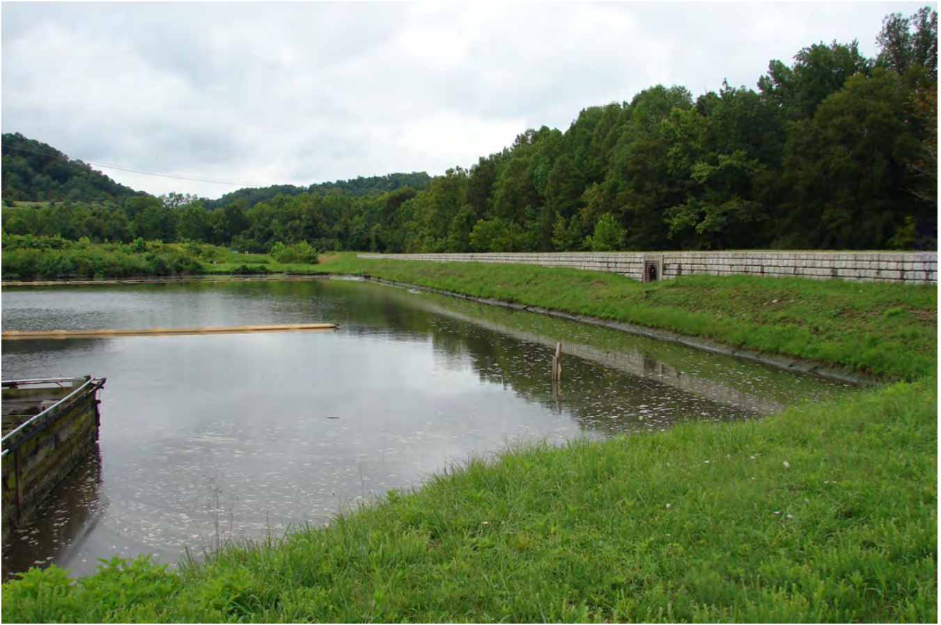
Photograph 6. Reclaim Pond and Upstream Slope.
