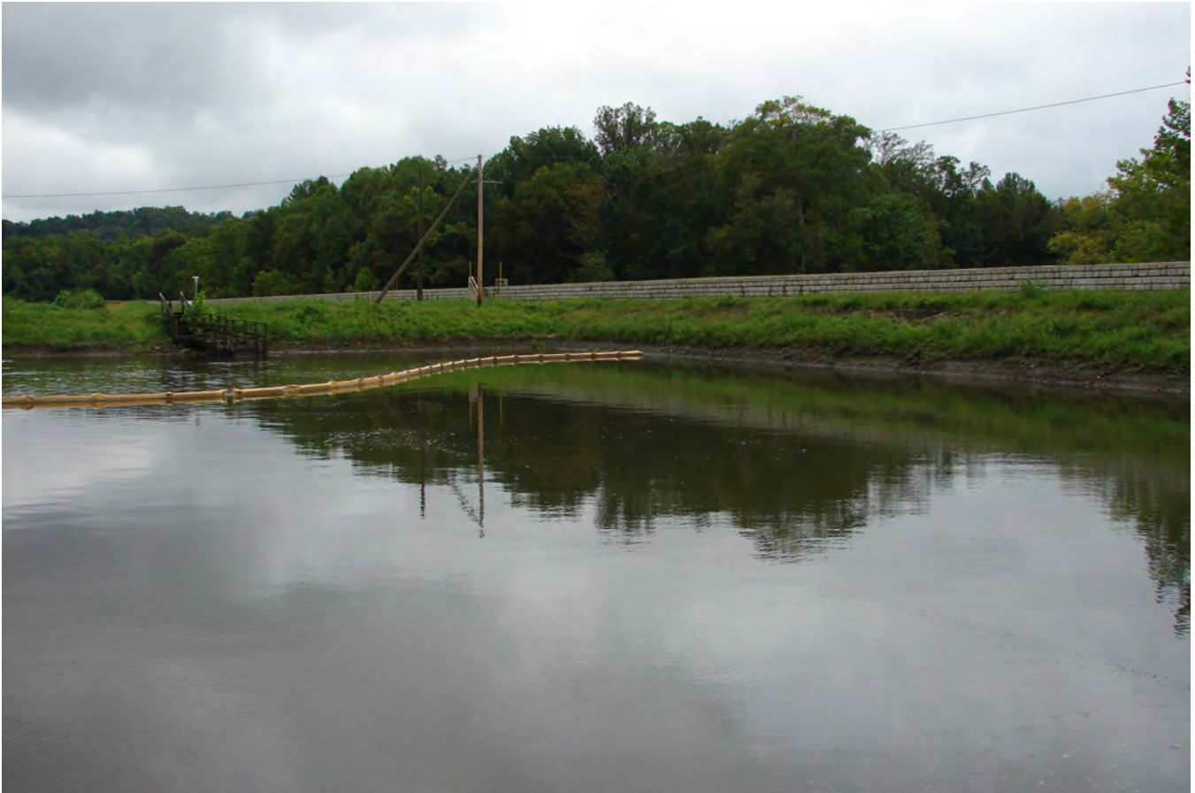
Photograph 5. Pond 1B and Upstream Slope.
