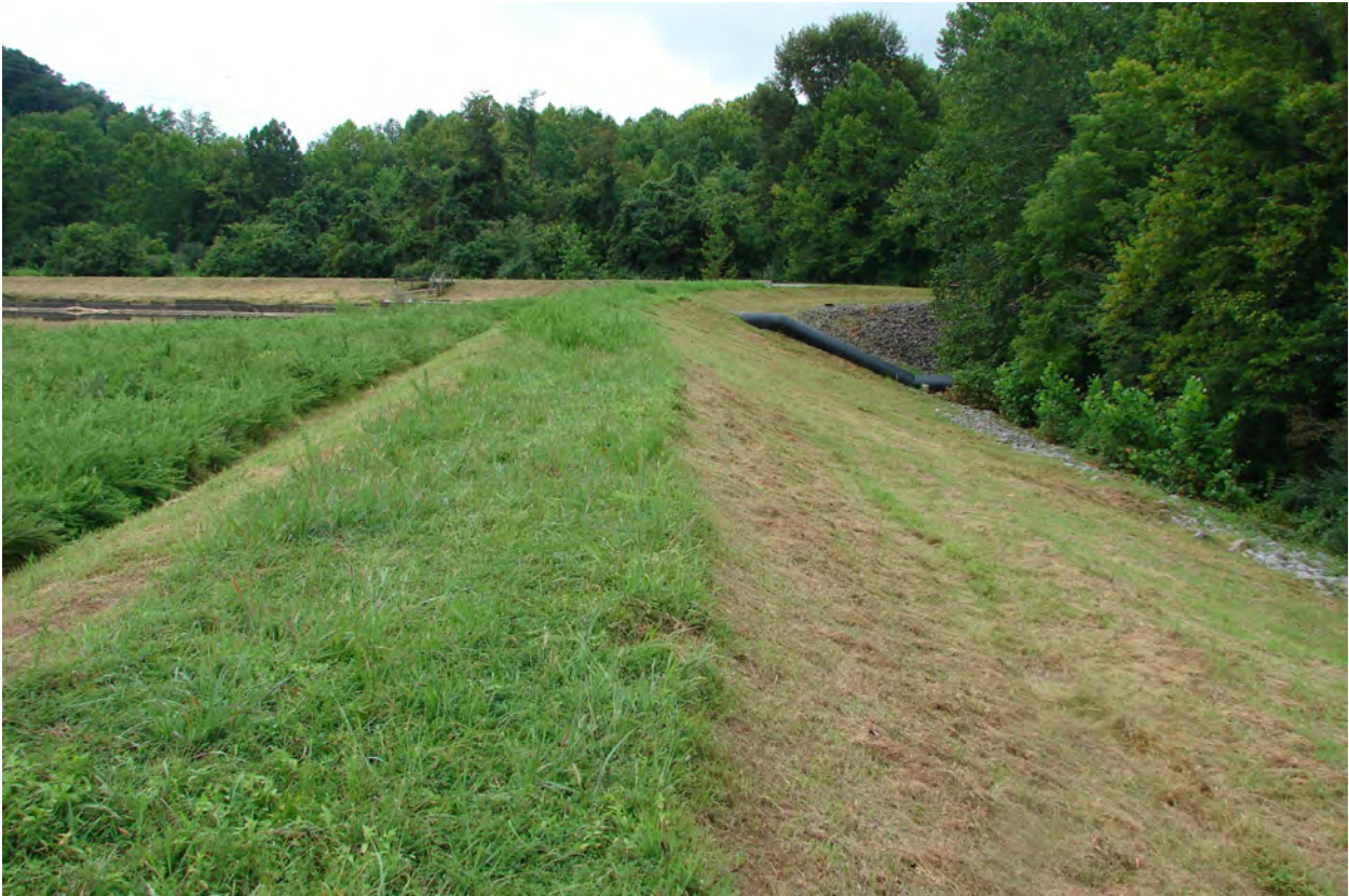
Photograph 1. Pond 1B Spillway Pipe and Downstream Slope
