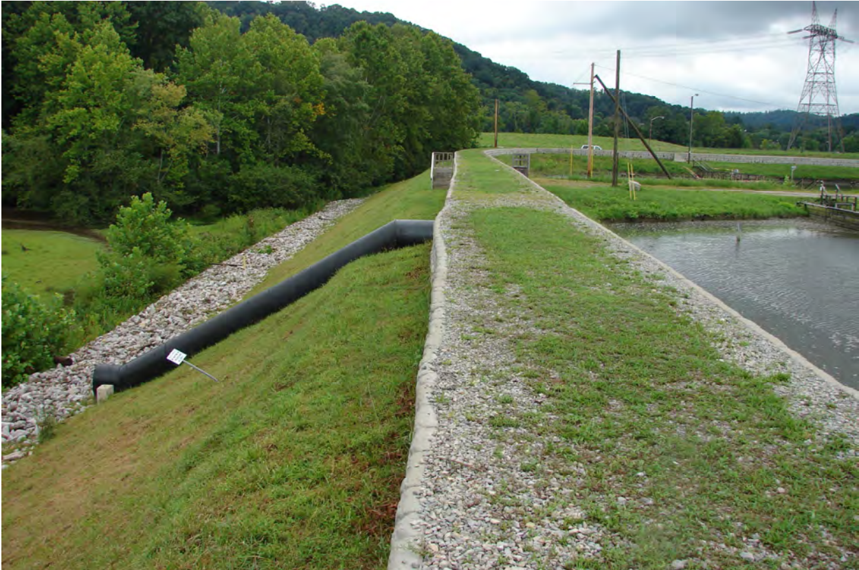
Photograph 2. Reclaim Pond Spillway Pipe and Downstream Slope.
